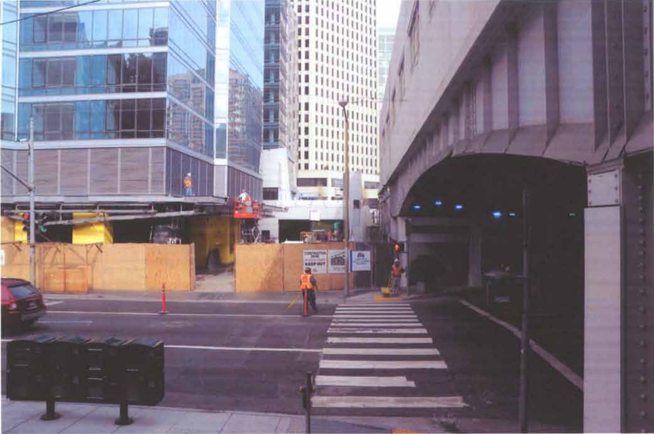
Transbay Terminal at Fremont View East
