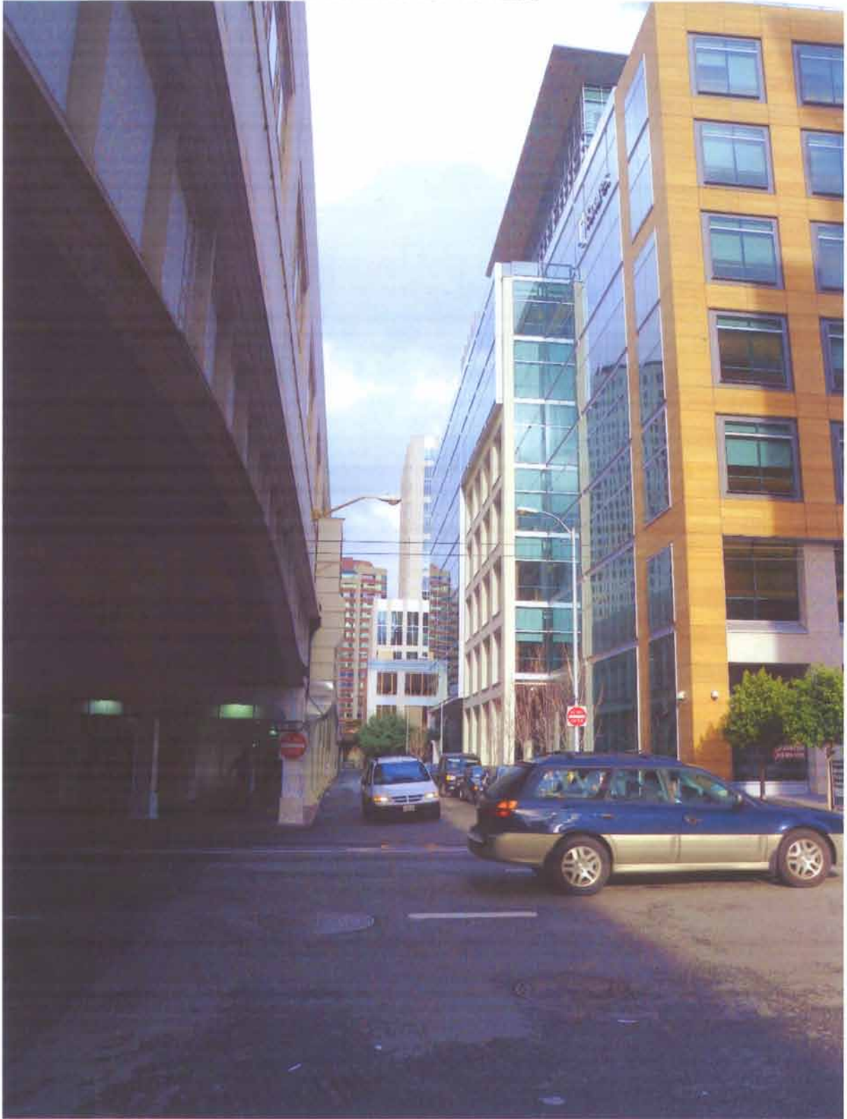
Natoma at First View East
