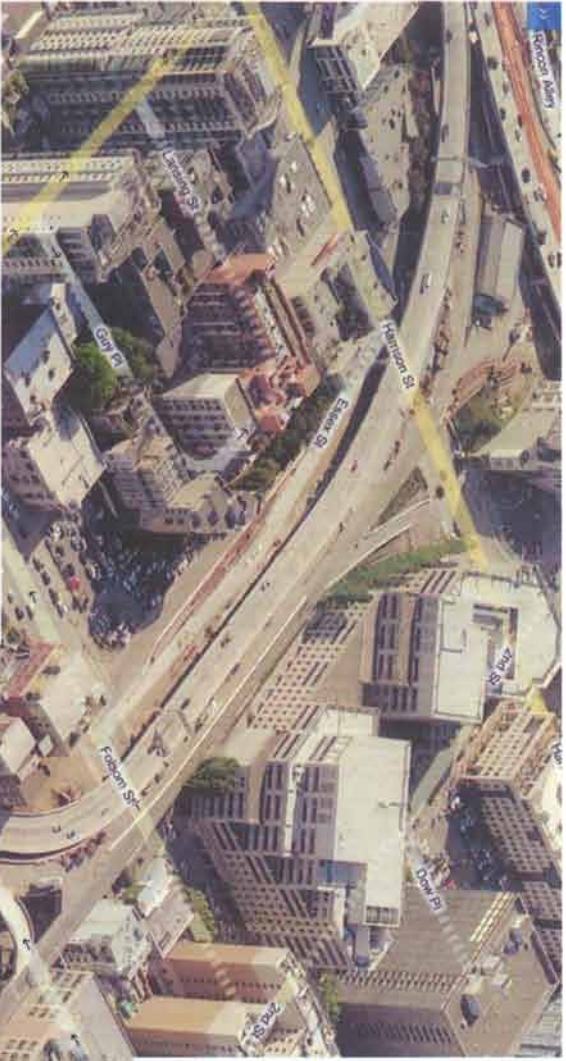
Existing Bus Ramps Overhead View
