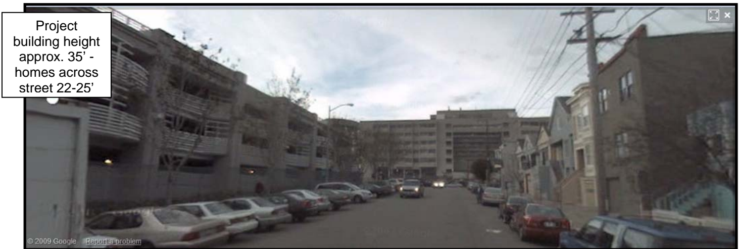
Viewing northerly along east side of project building on San Bruno Avenue.
