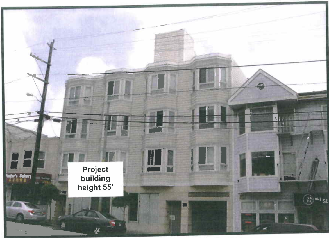
Viewing Southerly Toward Project Site from Opposite Side of Taraval.
