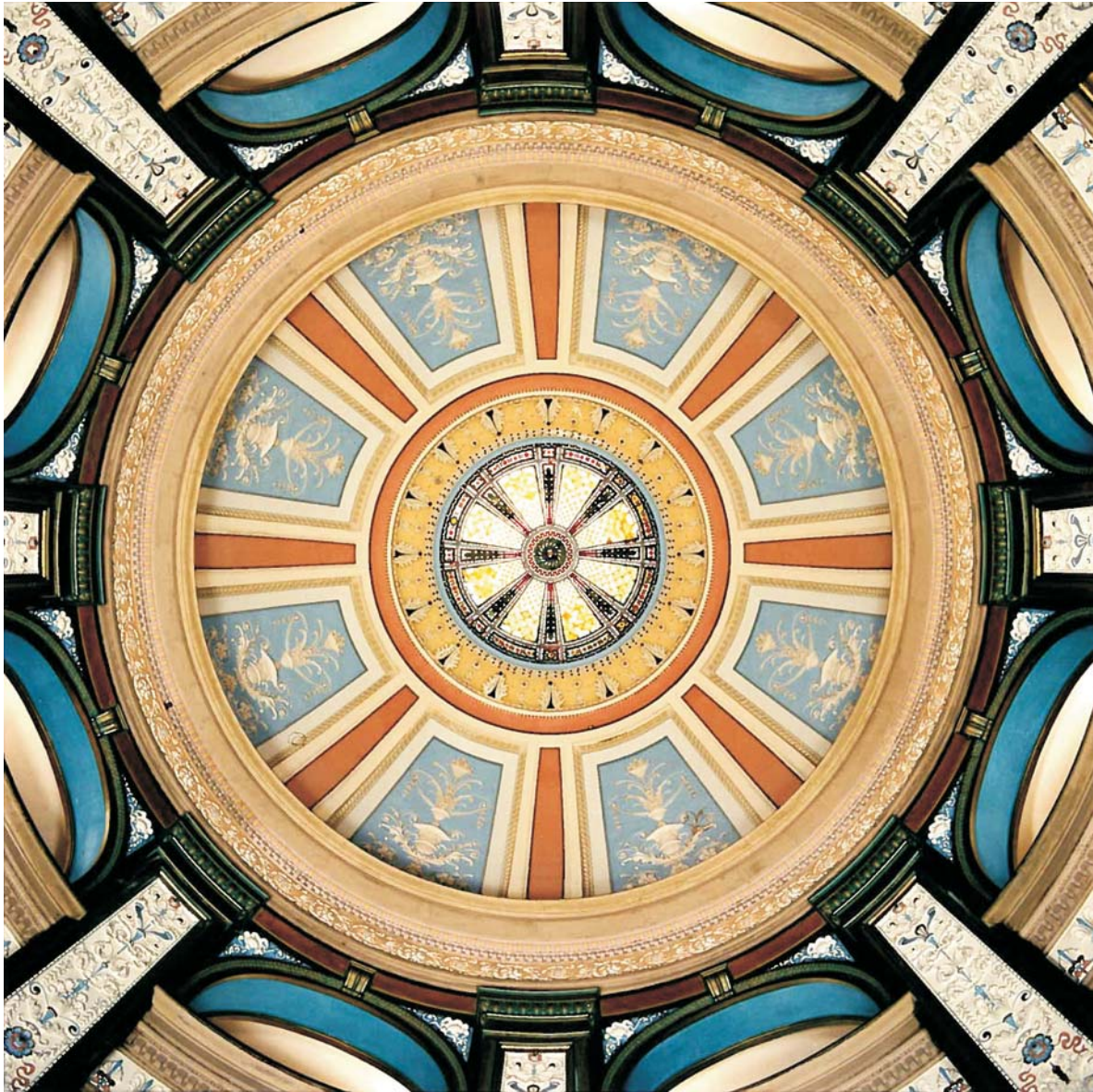
Columbarium Rotunda Dome & Skylight
