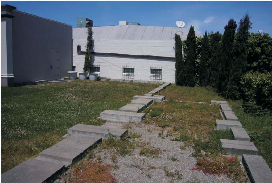
PHASE I NORTHEAST (view north): Proposed niche enclosure to replace previously approved niche wall footings & niche room and is to connect to the existing Support Building and hide back of Geary St. retail.
