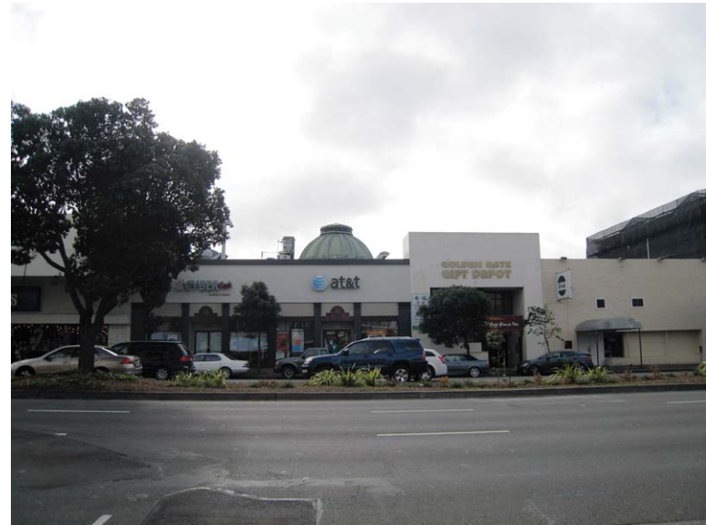
View of the project site from Geary Boulevard
