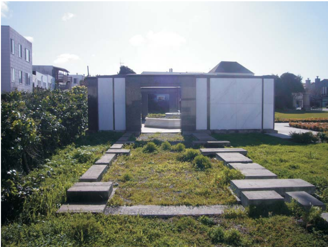
PHASE I NORTHEAST (view south): Proposed niche enclosure to replace previously approved niche wall footings, and to connect to Fountain Court.
