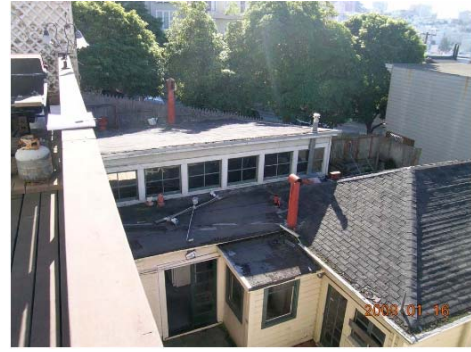
ROOF BETWEEN COTTAGE A + STUDIO
