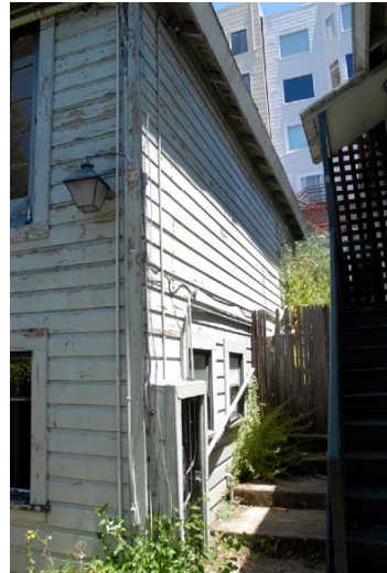
COTTAGE C South
