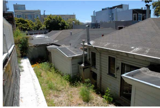
NON-CONTRIBUTING ADDITIONS @ COTTAGES B, C + D
