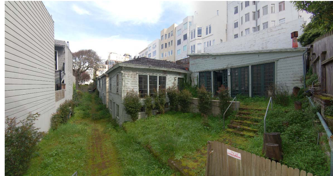
VIEW FROM INSIDE GATE
