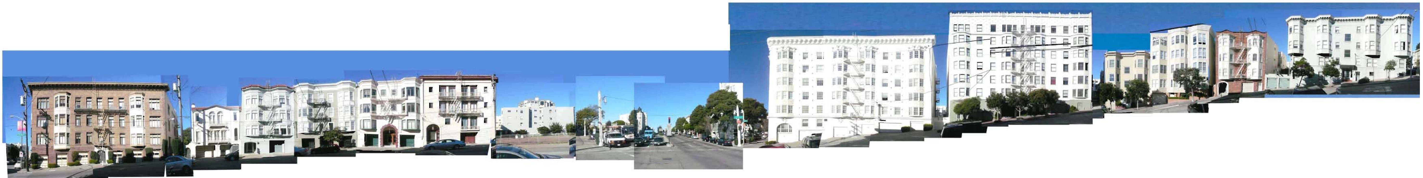
1 VIEW FACING NORTH ON FILBERT
