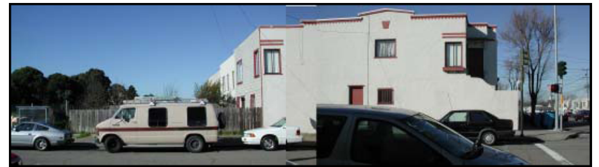
4 CAPITOL AVENUE WEST
