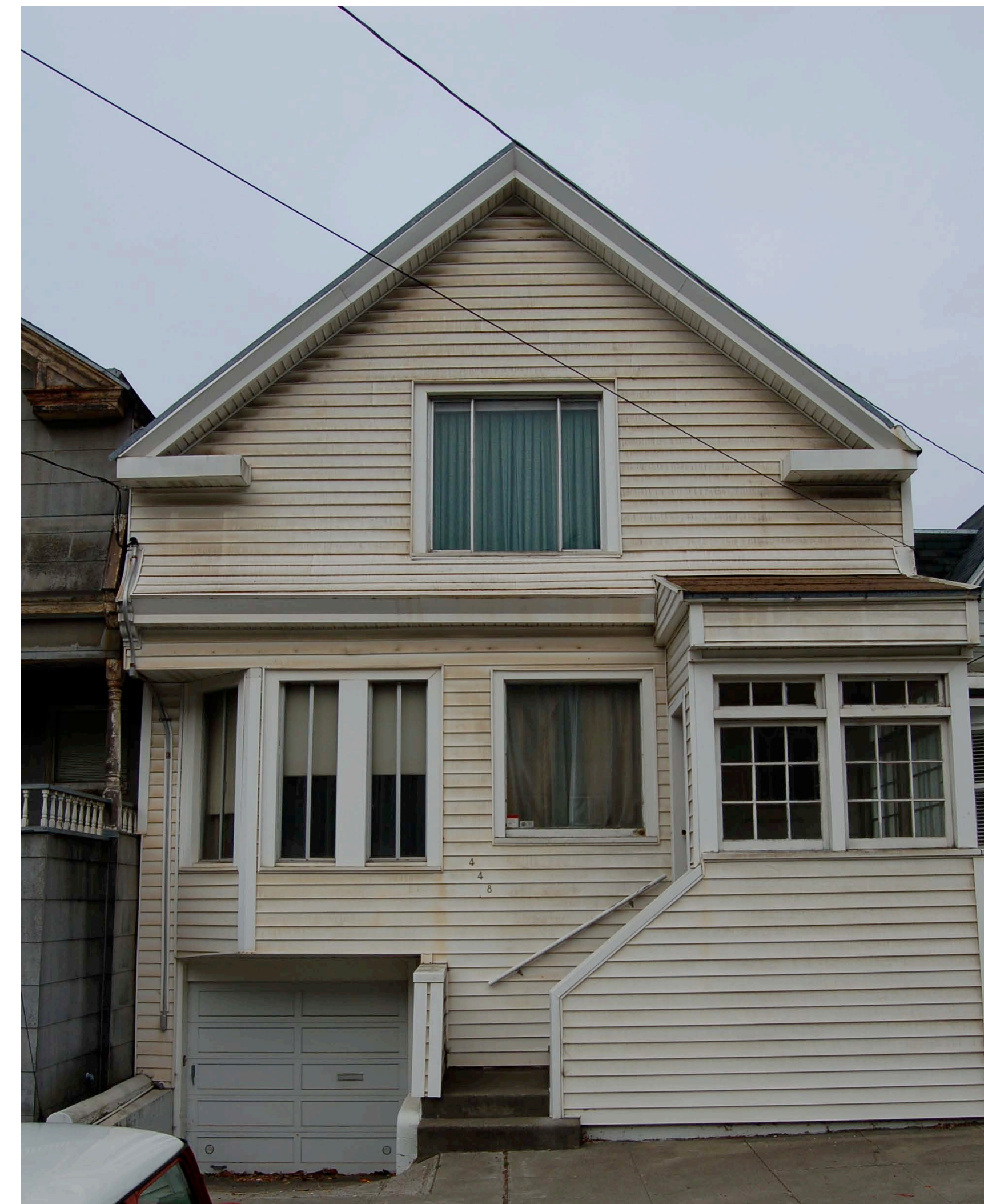
CLOSE UP OF EXISTING PROPERTY
