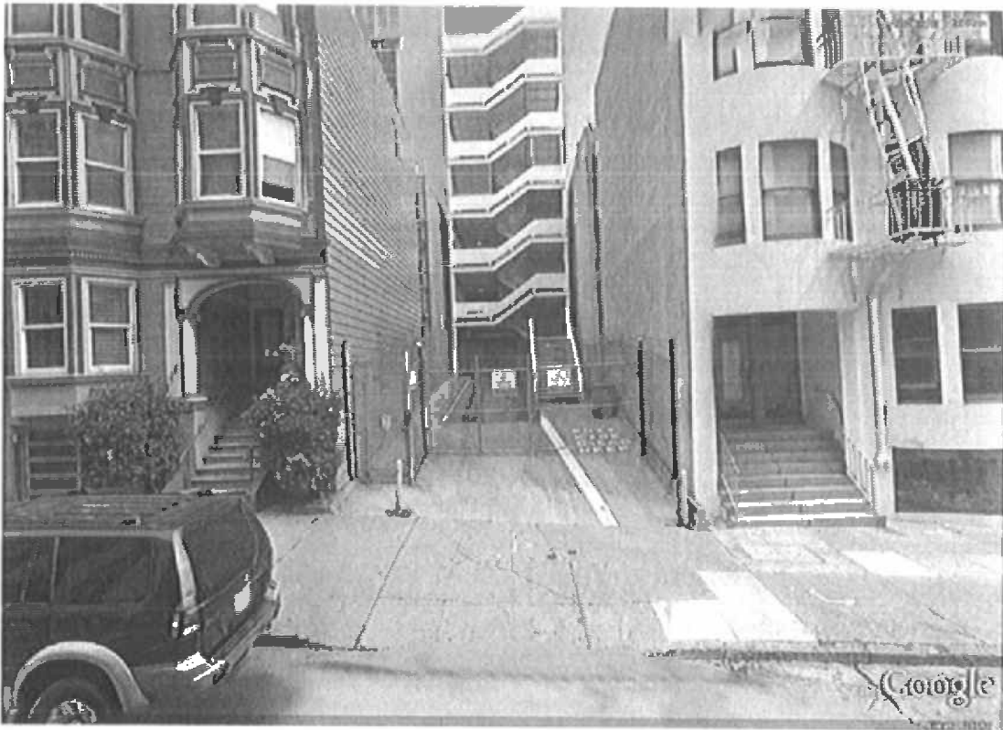
Pine Street Loading Dock
