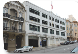
1234 Pine Street Parking Garage
