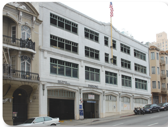
Pine Street Garage, Existing Signage
