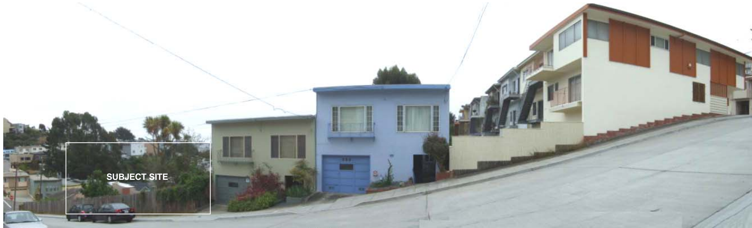
EXISTING SITE CONDITION - LOOKING FROM ACROSS LOS PALMOS
