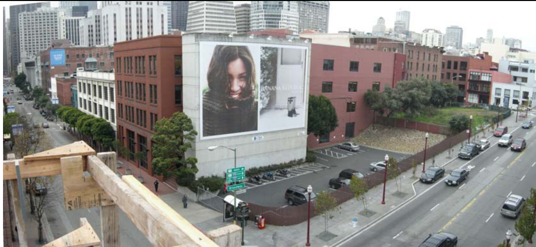
Panoramic View of Project Site
