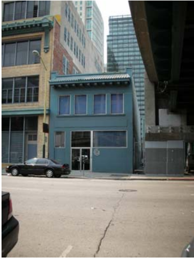
View from south side of Howard Street
