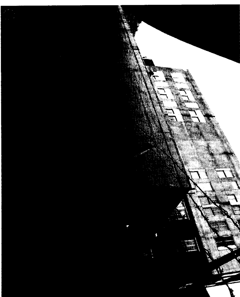
Photo "F" was taken from below the Transbay Loop, looking at the Northeast facade of the existing building on the project site.
