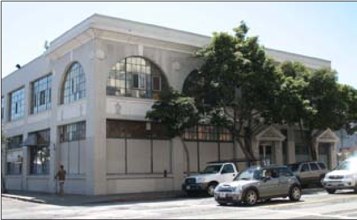
5 th Street Facade
