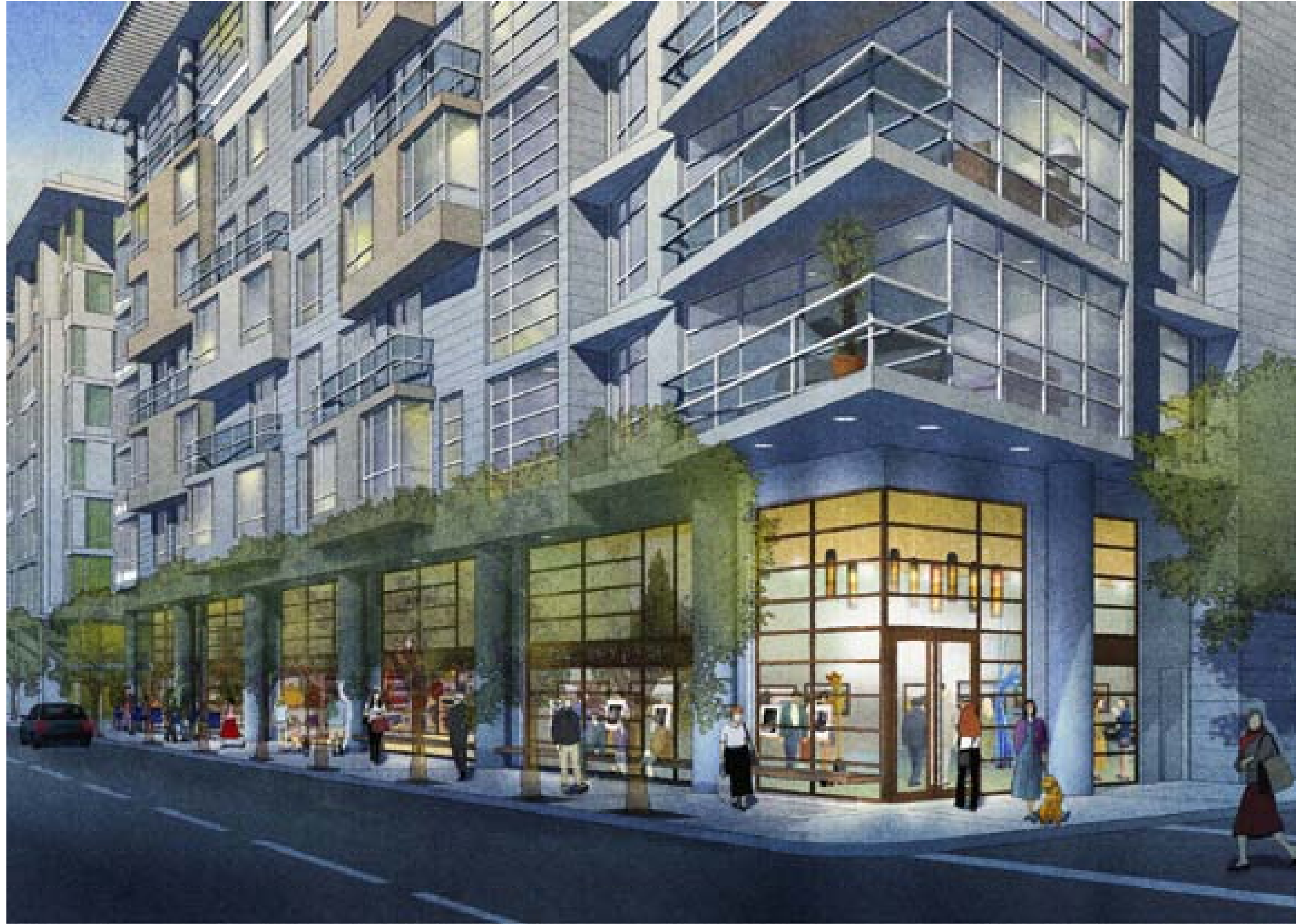
① 260 FIFTH STREET - CORNER OF TEHAMA AND FIFTH STREET SCALE: NTS
