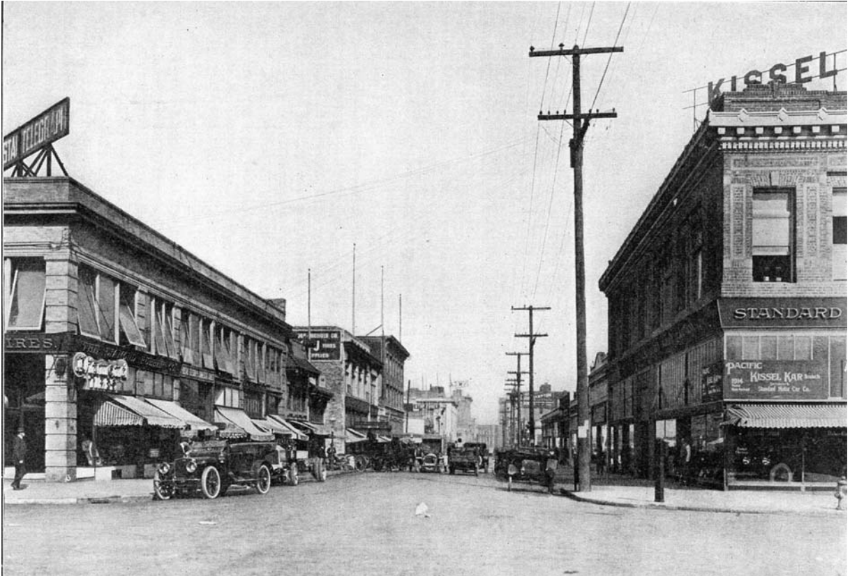
Looking east on Golden Gate Avenue from Van Ness in 1913. To the right is the building now numbered 550-590 Van Ness, then occupied by William L. Hughson's Standard Motor Car Co.
