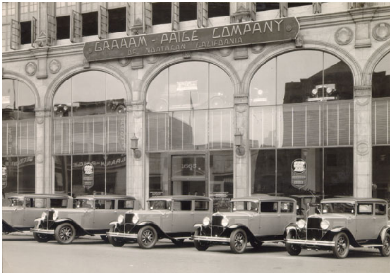
Two views of 1699 Van Ness Avenue, by Sylvain Schnaittacher. Its ground floor arcade hearkens to the Italian Renaissance. The northern three bays were built in 1919, and the southern two were added in 1923. Top photo: ca. 1953, SFPL Assessor's negatives. Bottom photo: ca. 1930, SFPL photo AAC-6822.
