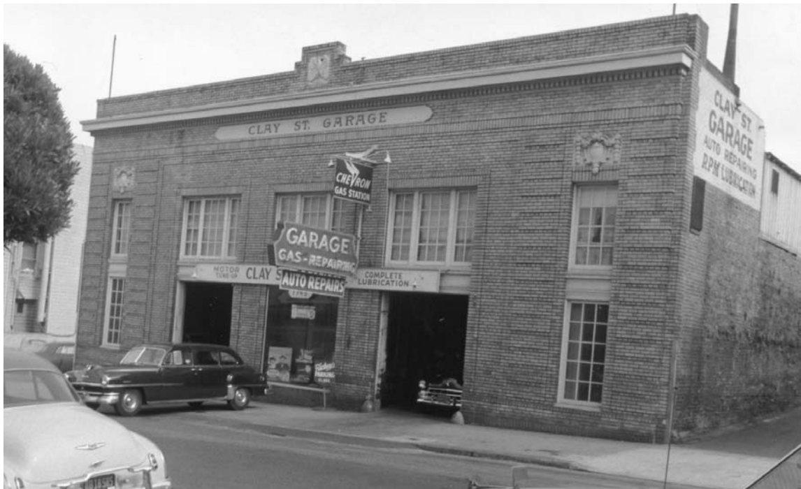
The Clay Street Garage, 1745 Clay Street, by architect James R. Miller, 1914. The window sash has been altered, but this brick masonry garage is otherwise intact. Photo: SFPL Assessor's negatives.
