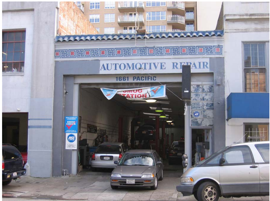
1661 Pacific Avenue, view of primary façade. Page & Turnbull, January 2008.
