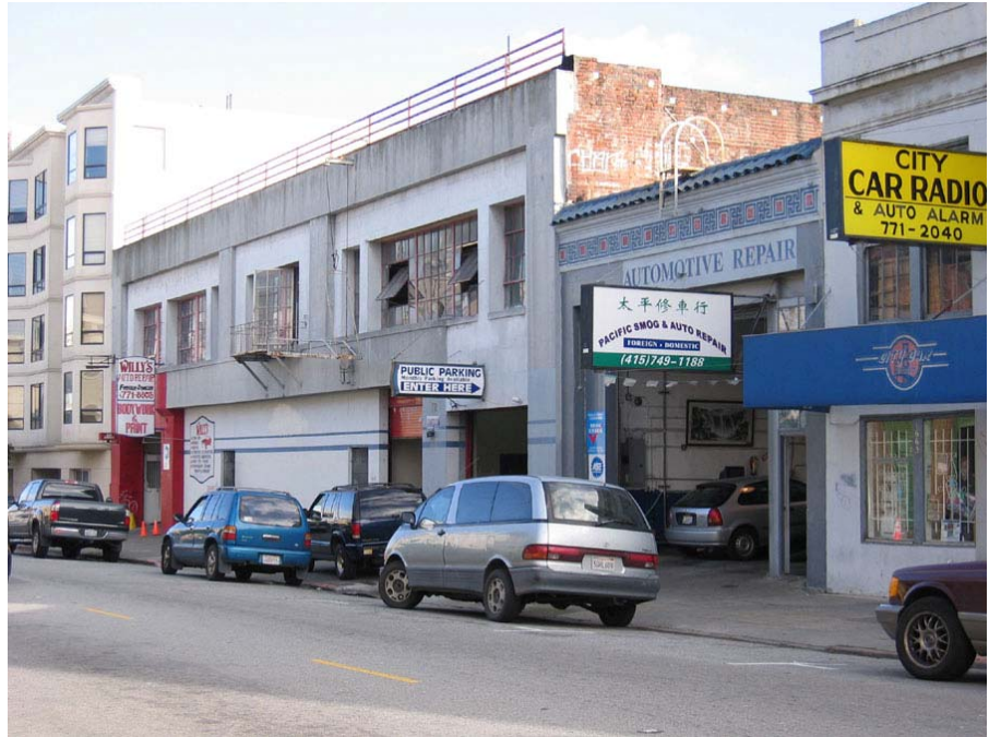
1661 Pacific Avenue, view east along Pacific Avenue. Page & Turnbull, January 2008.
