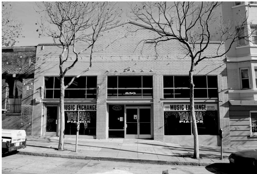
850 Van Ness Avenue (1919). Note the horizontal band which indicates where the pent roof used to be. Window sash have also been altered. This building was a used car salesroom from the time of its construction through at least 1964.
