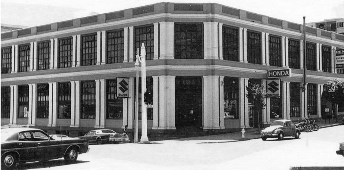
731-799 Van Ness Avenue. The first story of this reinforced concrete multiple-use building was built in 1916-1917 to designs of Willis Polk and Co., and the second story was added by the same firm in 1925, a year after Polk's death. Occupants through the early 1940s included auto repair shops, auto painting shops, and the Patrick J. Kelly Garage. Photo: Department of City Planning Van Ness Avenue Plan, 1980s.
