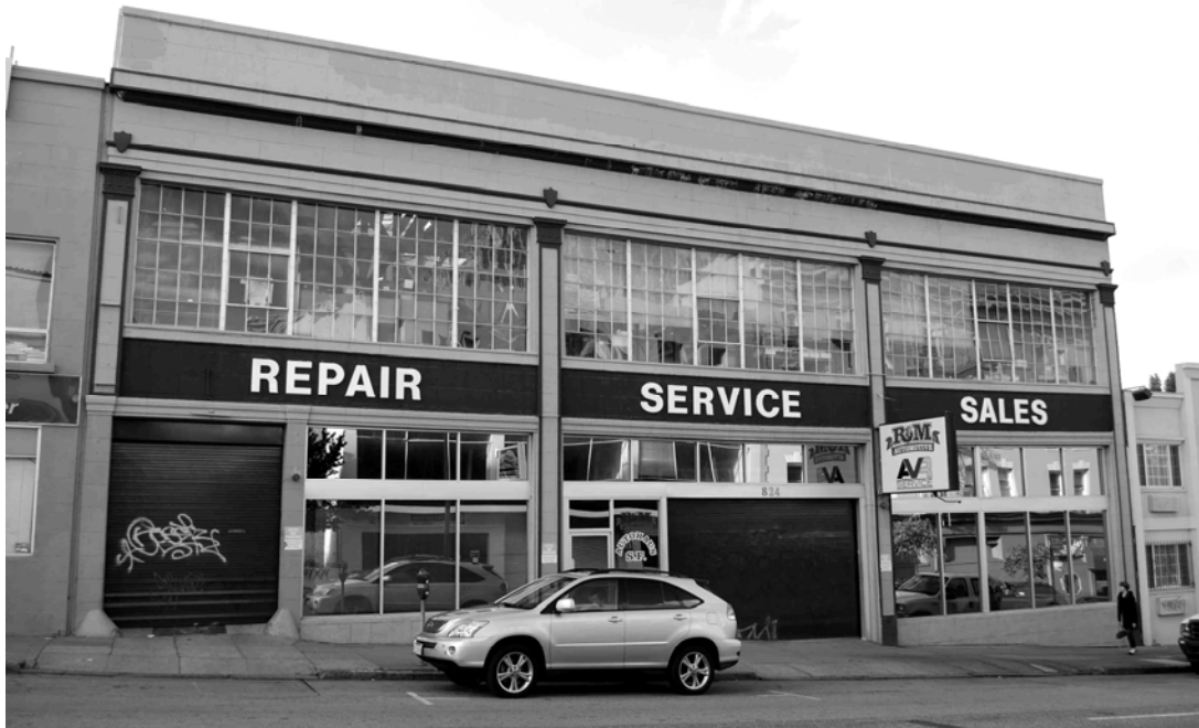
824 Ellis, a reinforced concrete auto repair shop with original steel sash. Built by the prolific builder William Helbing in 1920.
