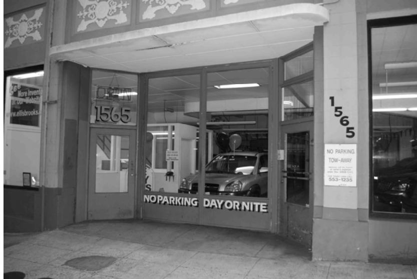
Paired vehicle doors with full-length glazing, at 1565 Bush Street. These are the last metal-framed vehicle doors in the Van Ness Avenue corridor.
