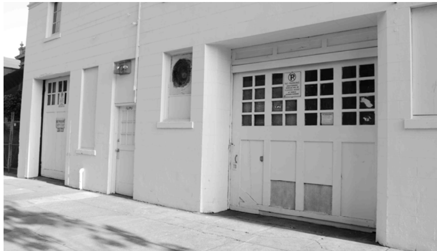
Two wooden doors at 1946-1960 Van Ness (on the Jackson Street side). One of these opens by raising, the other by sliding on rollers. Another building, at 731-799 Van Ness, also has two wooden vehicle doors.
