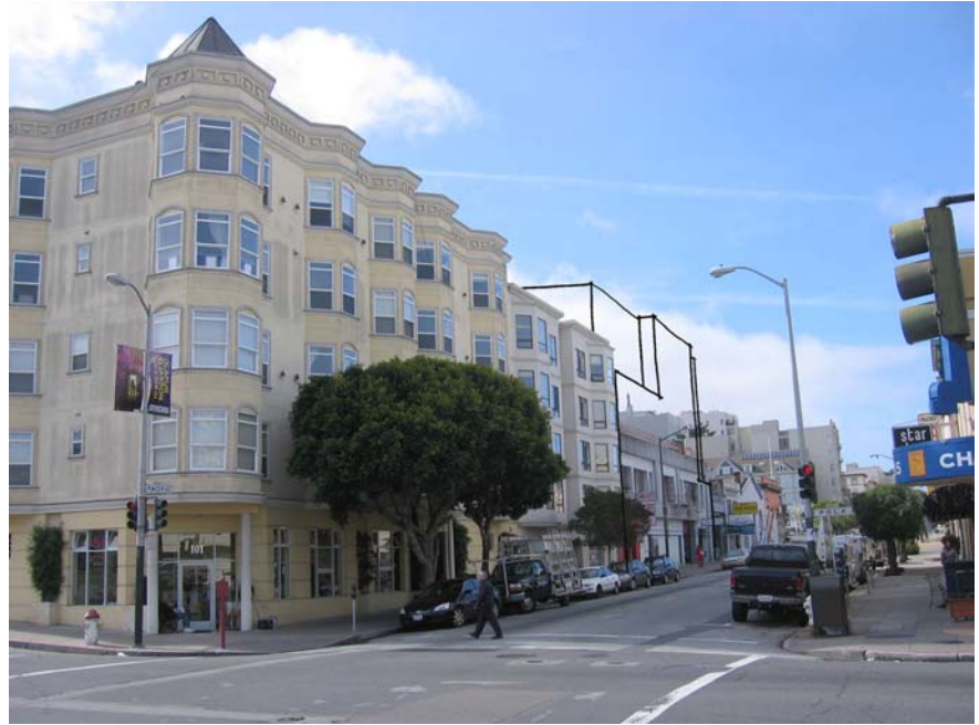
View west from Polk Street and Pacific Avenue, with massing of proposed project inserted
