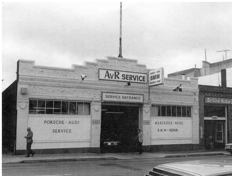
Four early garages, all made of brick, with symmetrical facades. In the top photo are 1) at right, the Alaska Garage, 1349 Larkin Street, by architects Ward and Blohme, 1909-1910; and 2) at left (partially visible), the Graystone Garage, 1335 Larkin, by John H. Powers, 1913-1914 (both extant). In the center photo is the Crown Garage, 1650 Jackson, 1910 (demolished). At bottom is the Pine Garage, 1461 Pine, 1911 (altered).
