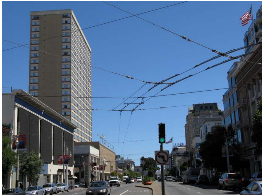
Van Ness Avenue at Sacramento Street. The eclectic mix of heights, uses, and architectural styles found within the “Auto Row” historic district is evident in this view.
