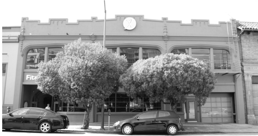
Kay's Garage, 1650-1660 Pacific Avenue. O'Brien Brothers, architects, 1921. This three-bay, two-story, reinforced concrete, Tudor Revival-style garage is similar to another garage by the same architects at 66 Page Street (1924). In this building, the original industrial steel sash windows have been replaced.
