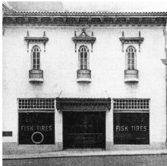
Fisk Tire Company, 1431 Van Ness. MacDonald and Applegarth, architects, 1911. Photo from a montage in the San Francisco Newsletter , Christmas number, 1913. Demolished.
