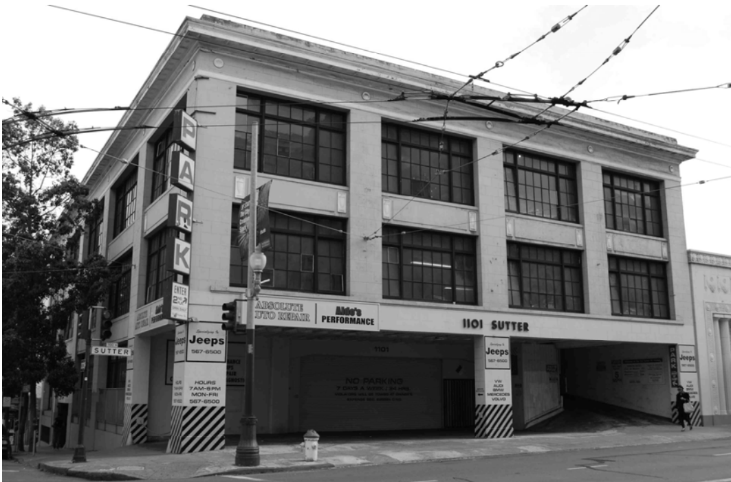
Heald's Engineering and Automobile School, 1101 Sutter Street. S. Heiman, architect, 1920. This is the last surviving example in the study area of this rare building type.
