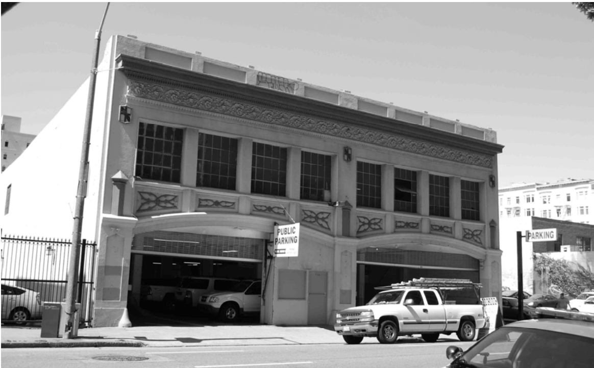
The Admiral Garage, 550 Turk Street. Joseph Pasqualetti, builder, 1924. It is two stories in height, two bays in width, and reinforced concrete in construction. Pasqualetti was a prolific builder of reinforced concrete buildings; here he employed both classical and Gothic decorative details.
