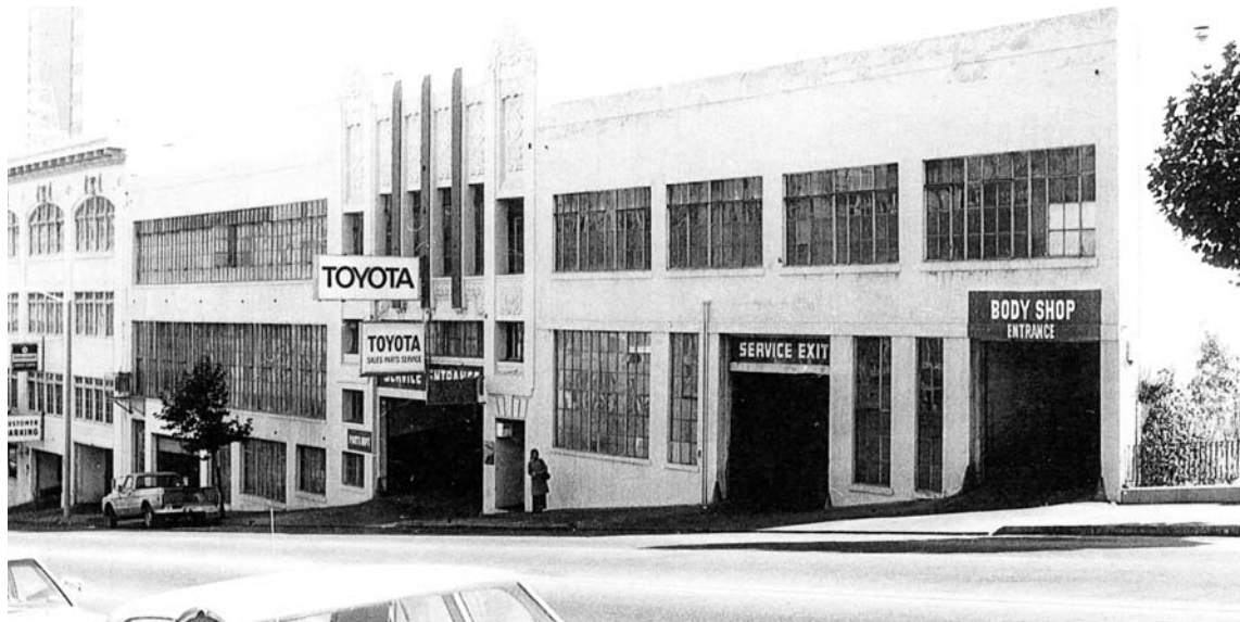
Hanni and Girerd's reinforced concrete auto repair shop, the largest in the study area, at 1765 California Street. The western wing was built first, in 1921, by architect T. Paterson Ross. The ornamental central pavilion and east wing were added in 1927 by Hyman and Appleton. This building's recent conversion to a grocery store retained the original steel sash windows.
