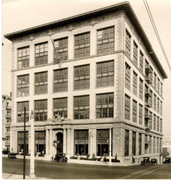
Don Lee's Cadillac showroom, 1000 Van Ness (extant). Weeks and Day, architects, 1921. (The interior is shown on the front cover of this report.) Photo: SFPL photo AAD-4657.
