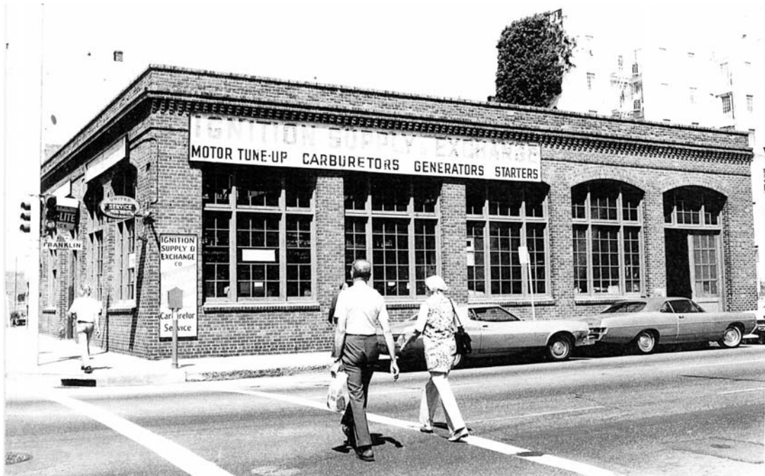
300 Grove Street, a brick auto repair shop with wooden window sash, built in 1920 to designs by architect A. Lacy Worswick.
