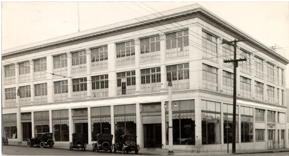
1700 Van Ness (MacDonald and Kahn, 1919; demolished) built as a showroom for Chandler and Cleveland autos. The skeletal construction was lightly decorated with classical ornament. SFPL photo AAD-4652.
