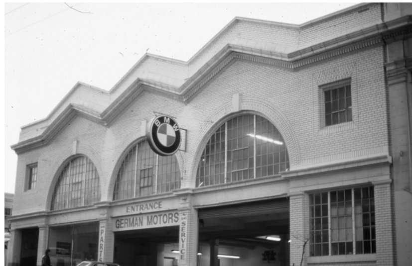
St. Francis Garage, 1240 Post Street, built in 1916 to designs by Sylvain Schnaittacher. Photo by William Kostura, 1983. This was a Class A steel-frame building with a brick front. It had the usual three-bay composition and industrial steel sash windows, but its zig-zag parapet and cornice were unique. This building and the adjacent Heald's College, also by Schnaittacher, were demolished in 1983.
