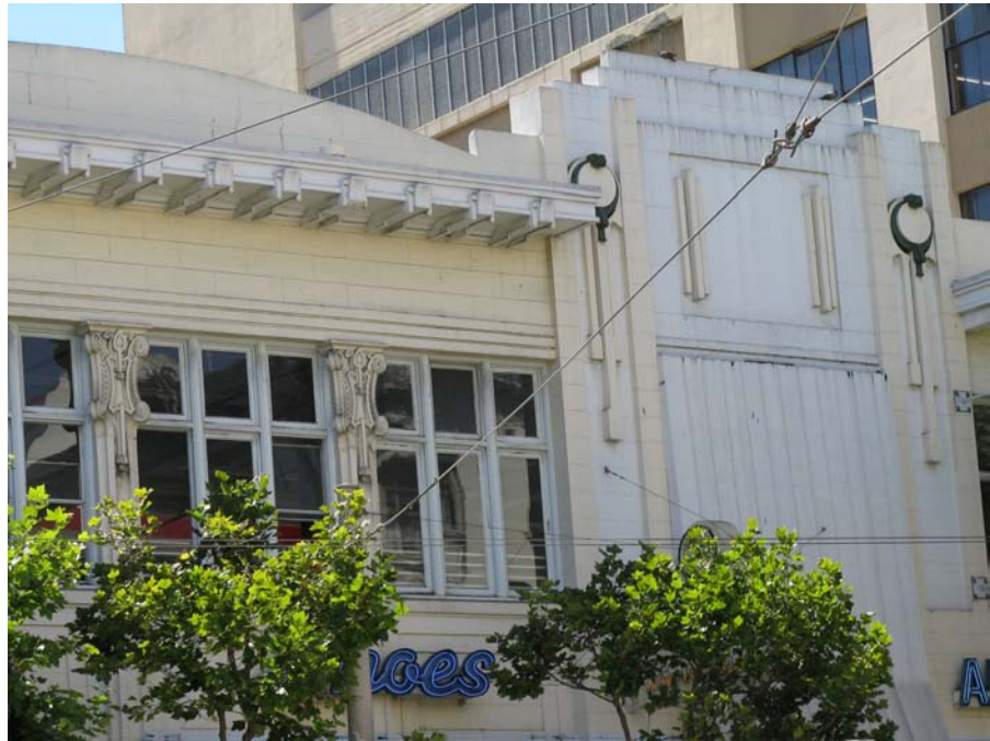
1301 Van Ness Avenue, at Sutter Street (1912). The cornice, windows, and ornament of this building are similar to the proposed design for 1645-1661 Pacific Avenue.
