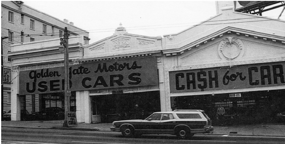
From left to right: 826 Van Ness (1918), 820 Van Ness (1920), and 810 Van Ness (1920). By mid-century, signage on used car salesrooms had become unsightly. All three of these buildings have been demolished. Photo from Department of City Planning 1976 survey.
