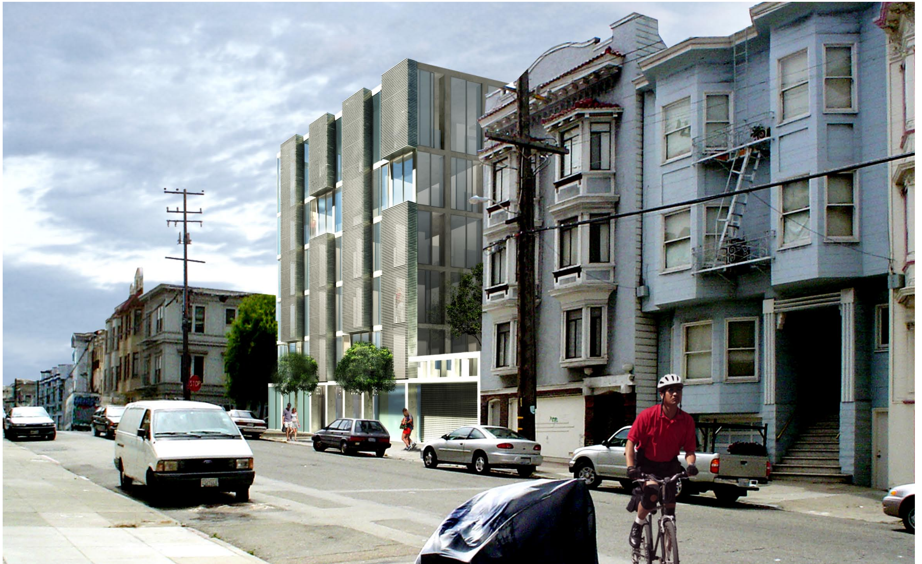
VIEW FROM LARKIN STREET
