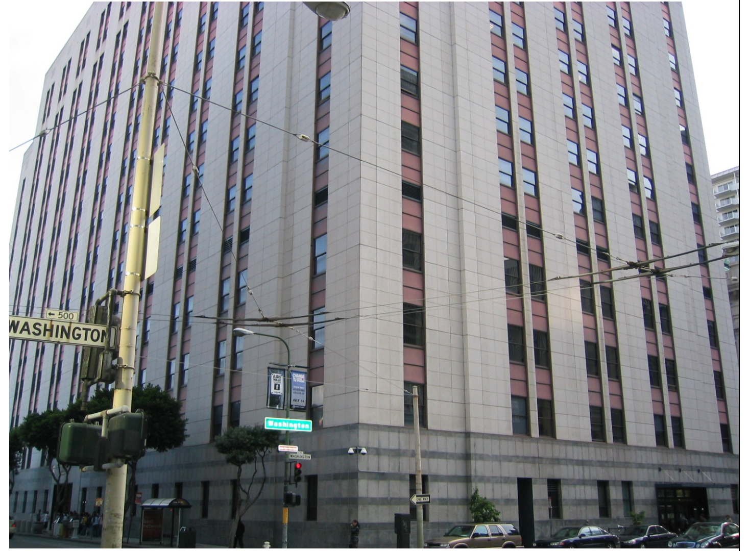
8. WASHINGTON STREET (LOOKING NORTHEAST OF PROJECT SITE)
