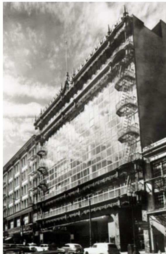
Hallidie Building, Date Unknown; source: San Francisco Public Library
