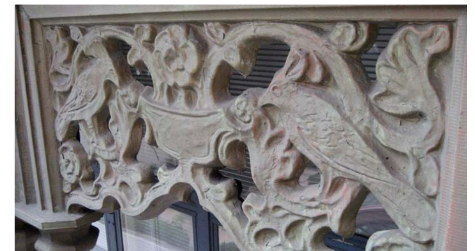
Decorative sheet metal below balconies
