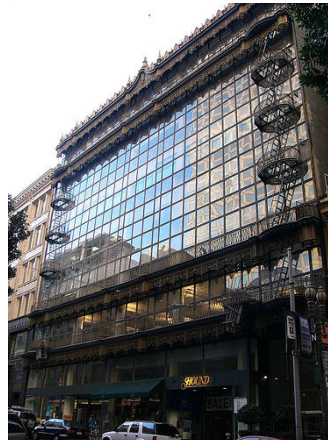
Existing building; source: http://www.docomomo-us.org
