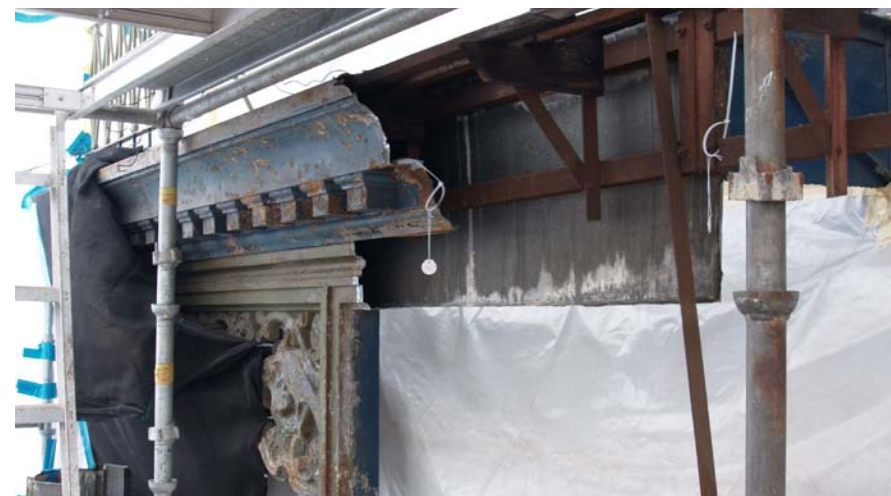
Cataloging and removing of decorative sheet metal
