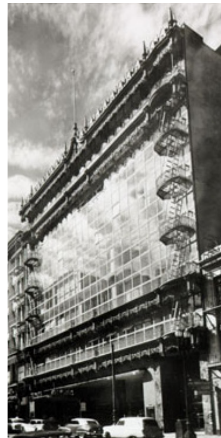
Hallidie Building, Date unknown; source: San Francisco Public Library
