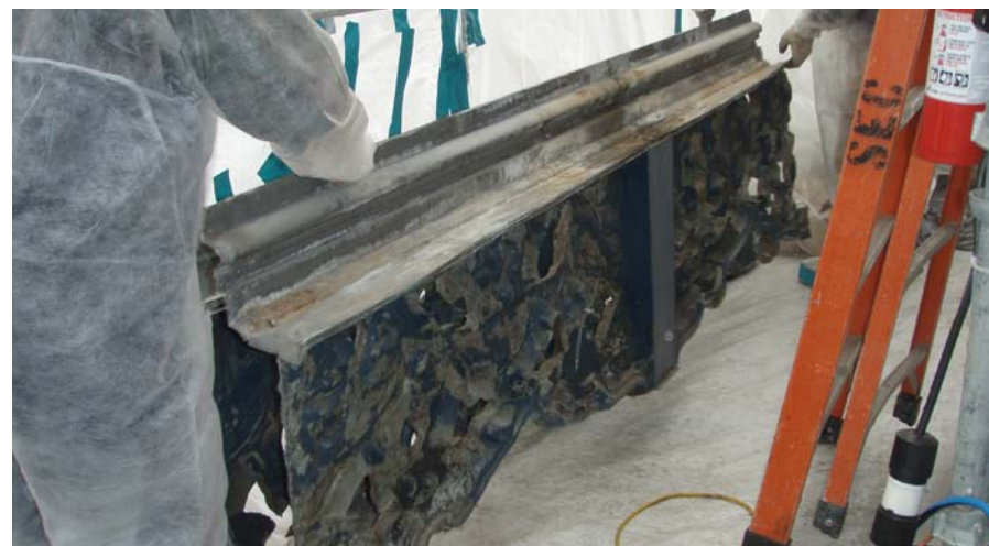
Decorative sheet metal is being removed where there are existing seams
