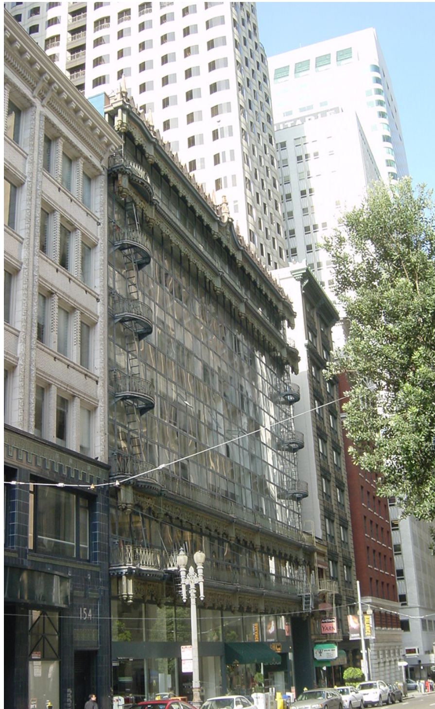
South facade; source: http://www.panoramio.com
