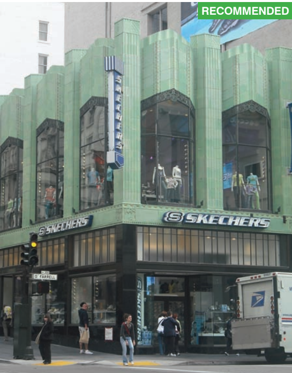
The rehabilitation project above preserved historic elements, such as the terra cotta tiles and cast iron framework. However, many other historic elements were missing, such as the transom windows and storefront pier material, were reconstructed based on historic documentation. It is common to use more than one approach in a rehabilitation project.
