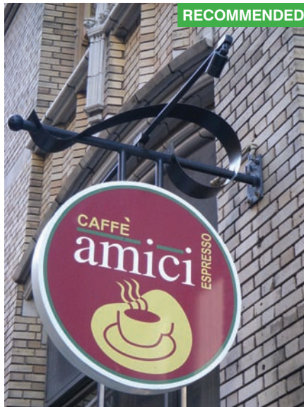
LEFT: This blade sign is placed at a height that relates well to the pedestrian scale of the street. It is low enough to read but high enough not to block the public right-of-way. It is also attached to a contemporary storefront so not to damage the building's historic elements.
