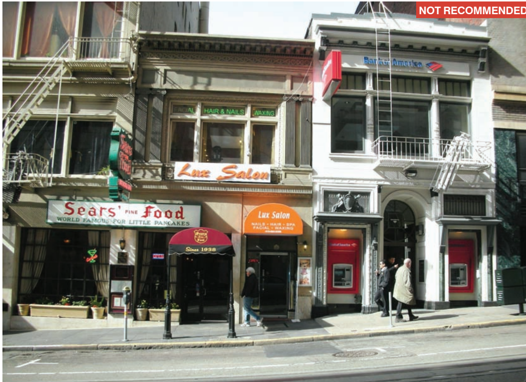
The purpose of this document is to avoid overwhelming and confusing streetscapes as indicated above. In this example the signs and awnings do not correspond well to the appropriate business, extend over bays and storefronts, and they obscure the character-defining features of the buildings.
