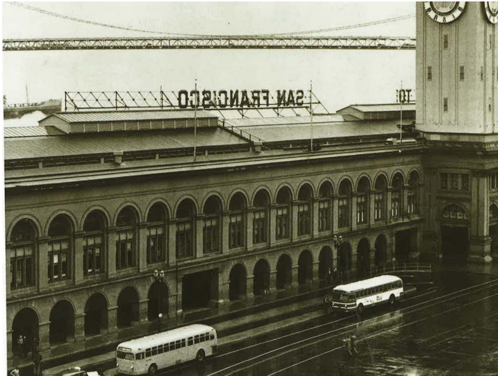
View of the north arcade in the 1940s
