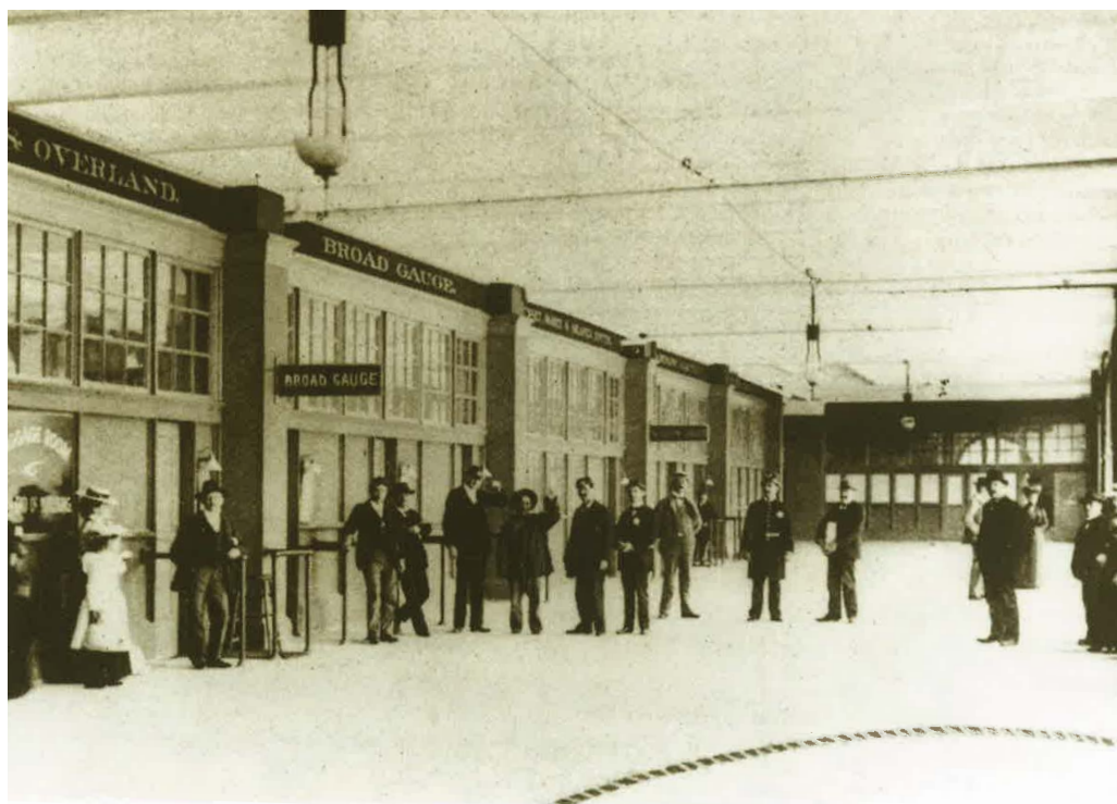
View of the south arcade when it was used for ticketing, c. 1904
