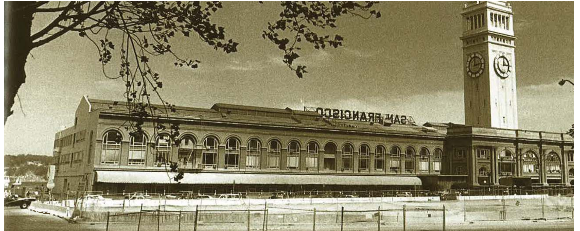
View of the north arcade after it was infilled in the 1950s
