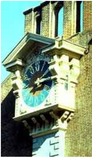
In the reconstruction of the clock tower at Independence Hall, the substitute materials used were cast stone and wood with fiberglass and polyester bronze ornamentation. Photo: NPS files.
