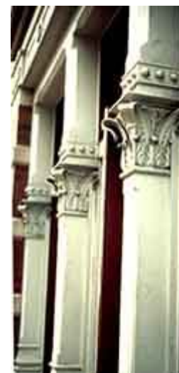
Cast aluminum has been used as a replacement material for cast iron. Photo: NPS files.
