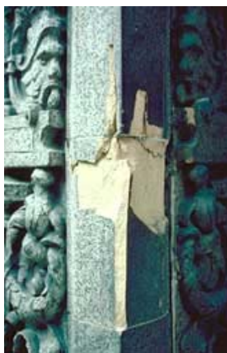
The damage shown here is the result of direct live load on a mid-rise building. The steel frame has settled and shifted the weight onto the exterior terra-cotta cladding, resulting in rupturing of the material. Photo: NPS files.
