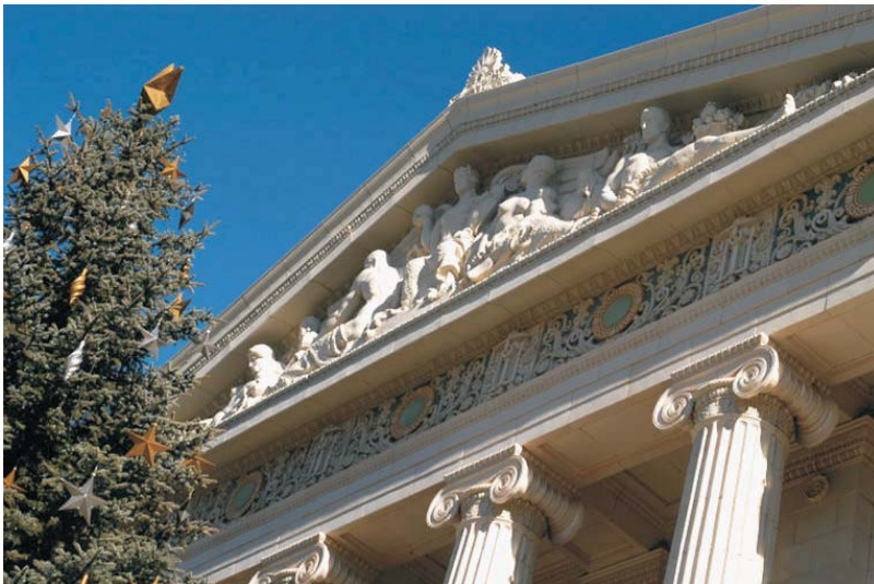
PHOTO: Three custom colors of Aquathane UA210 E were used on extensive terra cotta glaze repairs at this Historic Register site.
