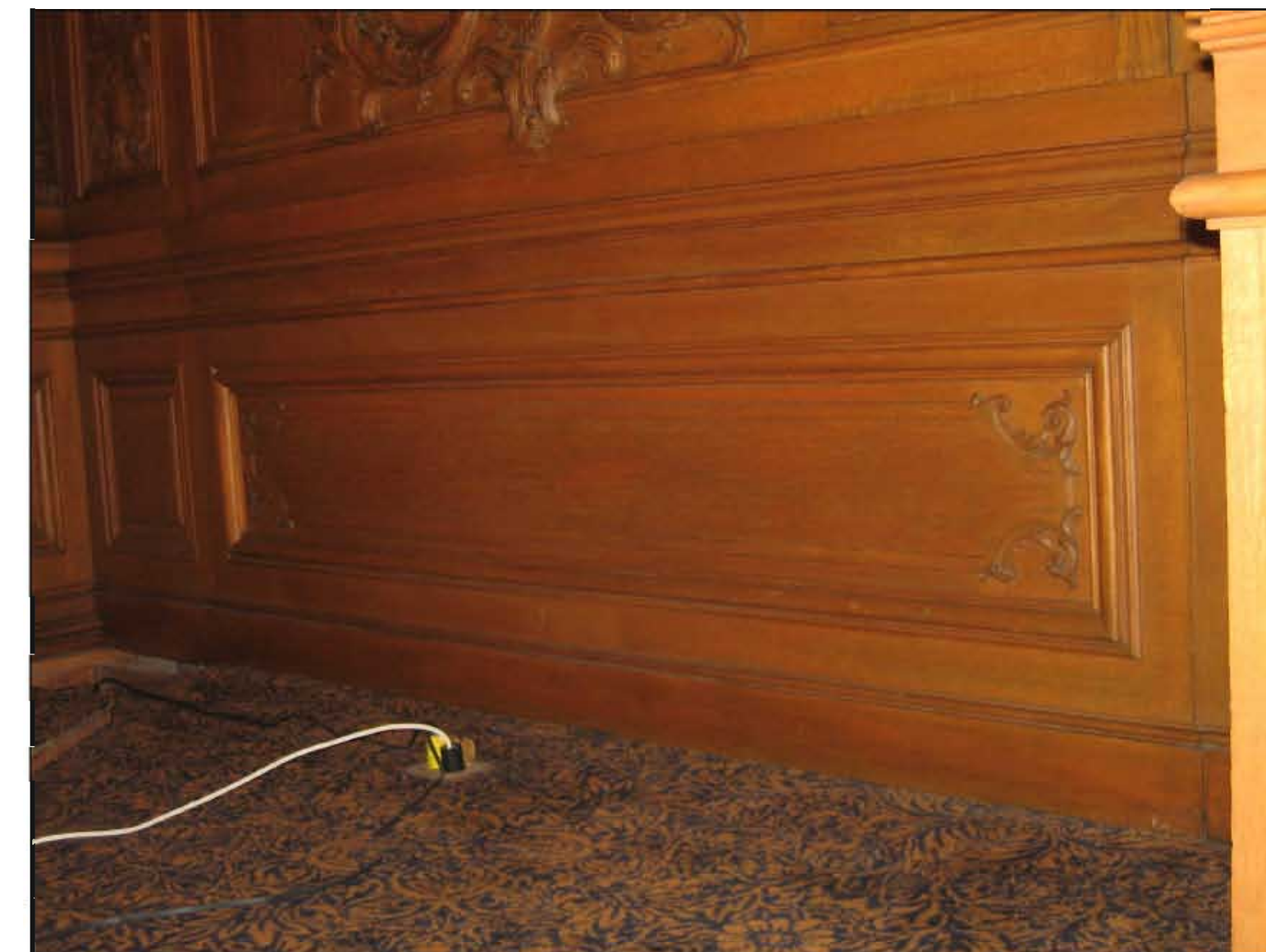
3 SOUTH WALL- Wood Wainscot, Looking East SCALE: NTS
