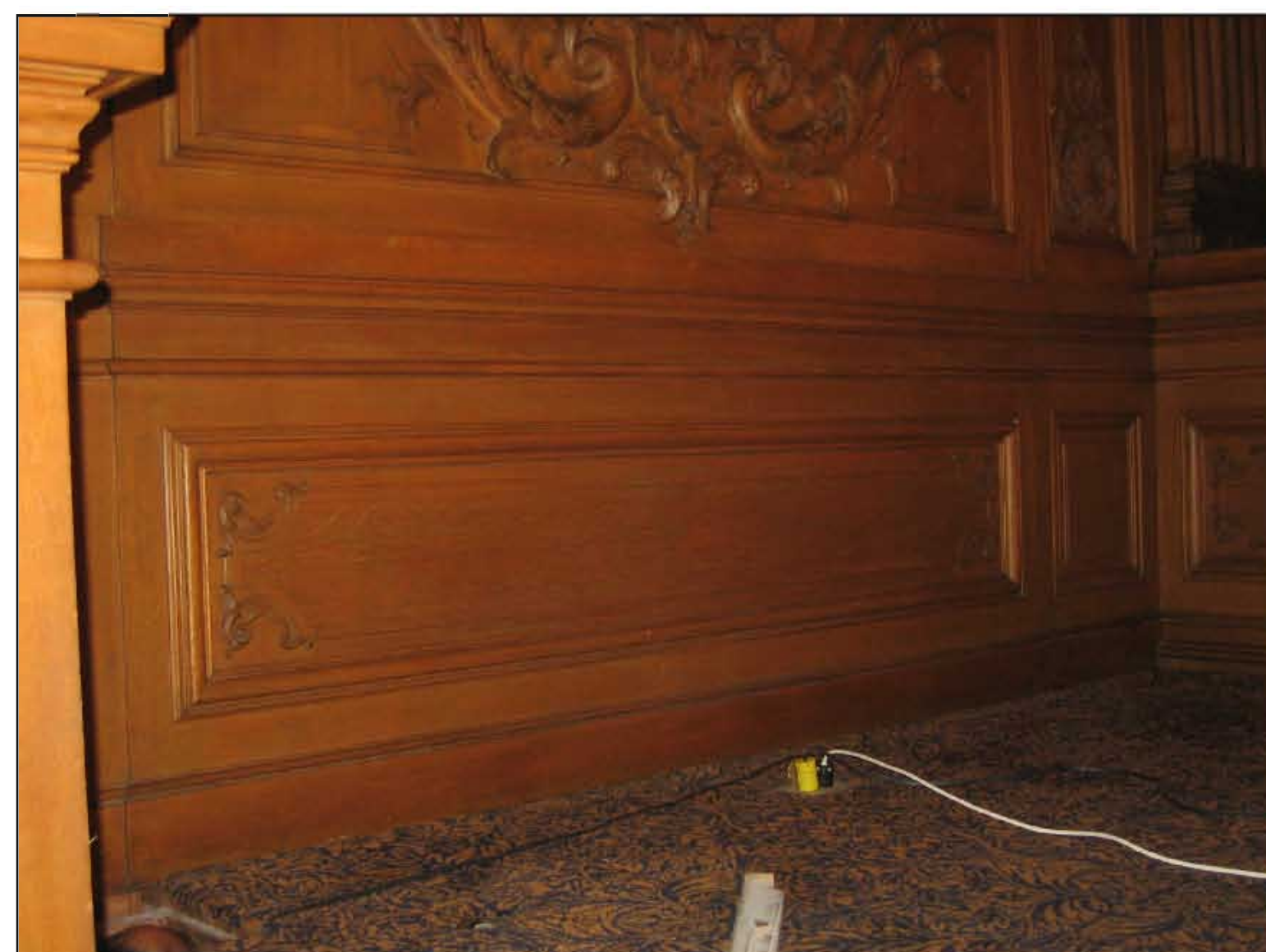
8 SOUTH WALL- Wood Wainscot, Looking West SCALE: NTS
