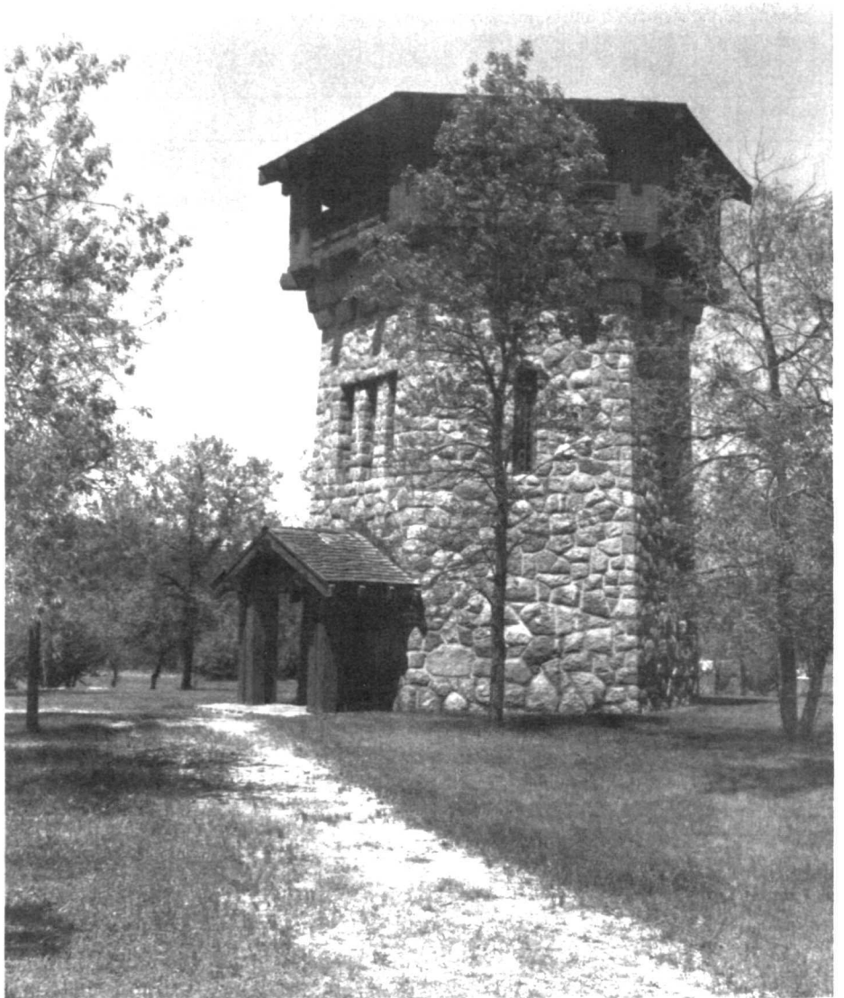
The 1939 water tower is a contributing building in the National Register of Historic Places nomination of Lake Bronson State Park in Kittson County, Minnesota. The eligibility of the park was justified for its association with the Minnesota State Park CCC/WPA/Rustic Style Historic Resources multiple property submission. The historic resources of Lake Bronson State Park are significant as "outstanding examples of rustic style split stone construction." (Rolf T. Anderson)
