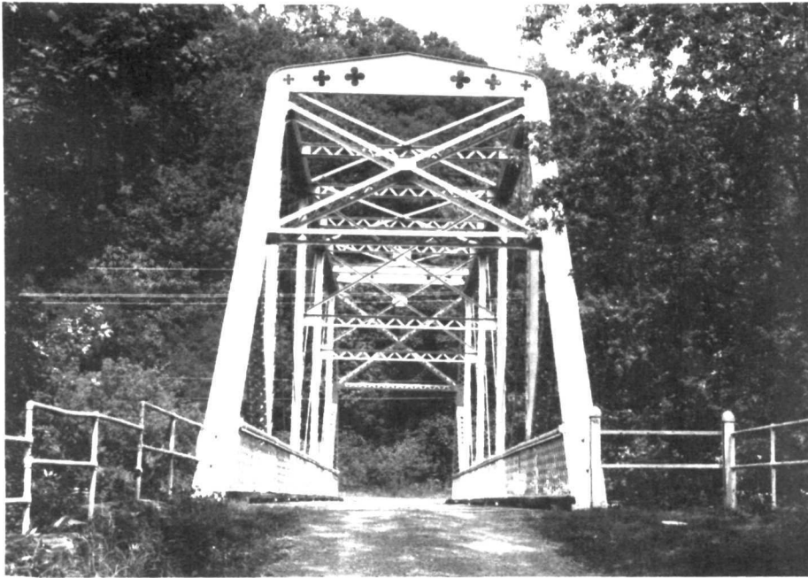
The 1898 Birmingham Bridge was nominated to the National Register of Historic Places as part of the Industrial Resources of Huntingdon County, Pennsylvania multiple property submission. Located in Birmingham, it is significant as "a fine example of one of the county's less than ten remaining pin-connected Pratt through truss bridges built in the late 1800s." (Nancy Shedd )
