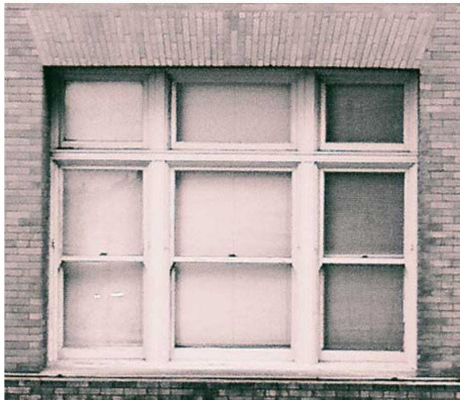
EXISTING WINDOW AT 2ND FLOOR (MARKET, 7TH AND STEVENSON STREET)
