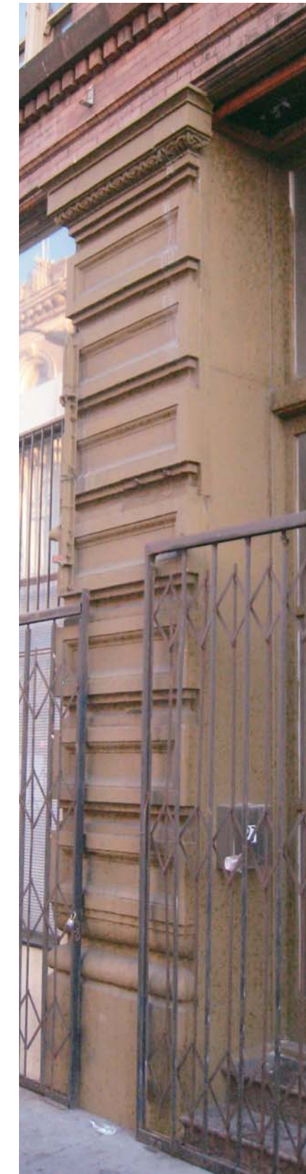
EXISTING PILASTERS PHOTOS 37
