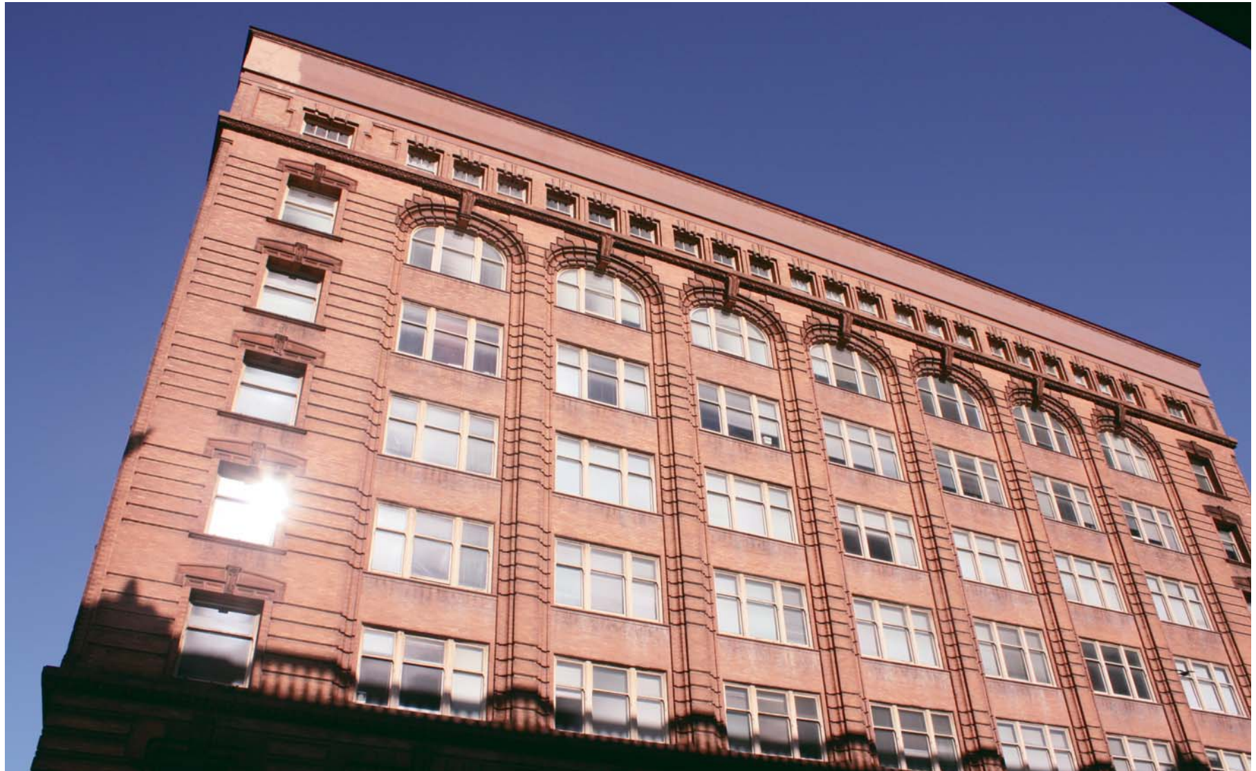
View K - 7TH STREET AT UPPER FACADE
