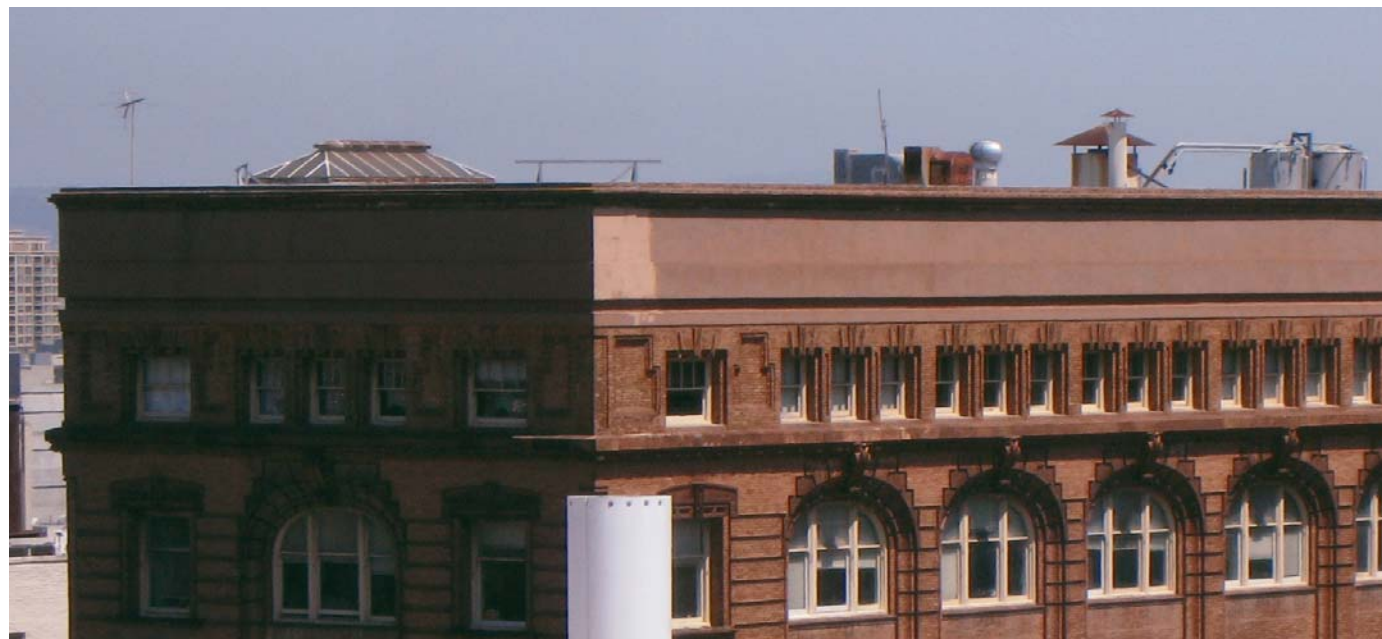
EXISTING CORNICE CONDITION
