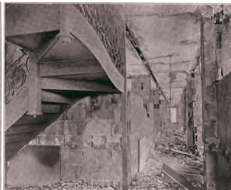
GRANT BUILDING. Typical view showing the damage to the hollow-tile column protection and the failure of the hollow-tile partitions. The Roebling concrete floors and wire lath and plaster ceilings are in good condition throughout.
