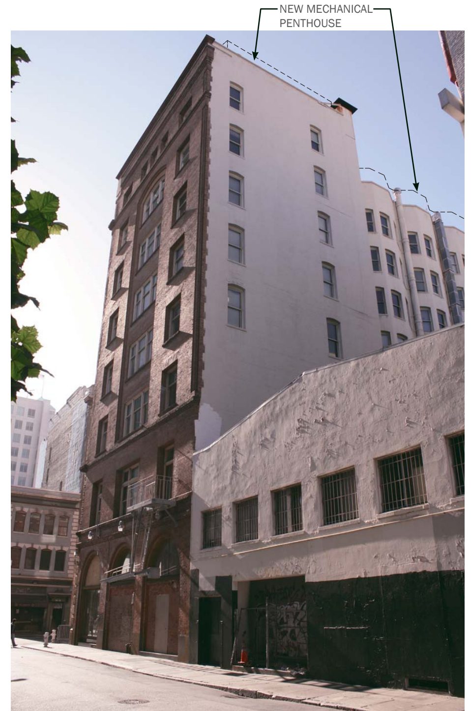
View G - VIEW FROM STEVENSON STREET (SEE PAGE 6 FOR VIEW POINT)
