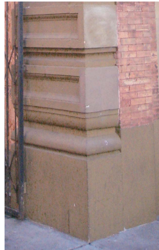
EXISTING PILASTERS AT THE CORNER OF 7TH AND STEVENSON STREET
