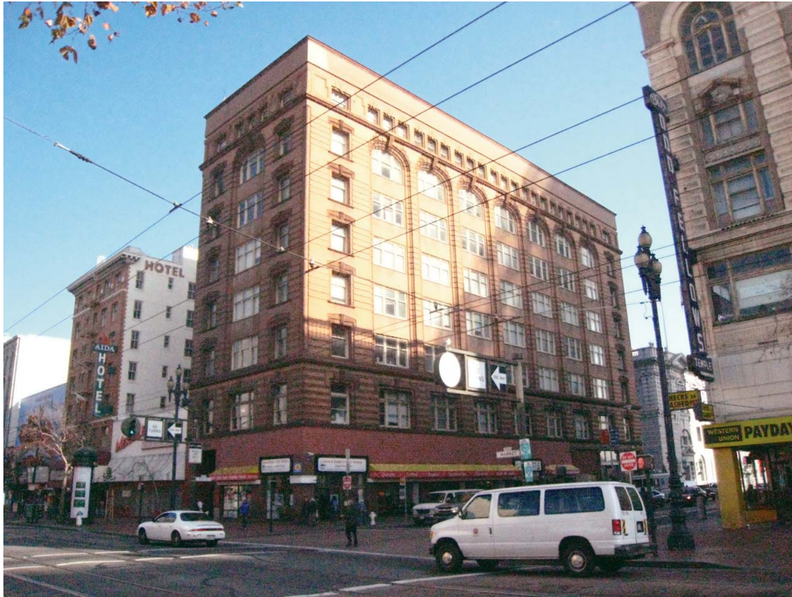
View A VIEW TODAY ALONG MARKET AT 7TH STREET (NORTHWEST CORNER)
