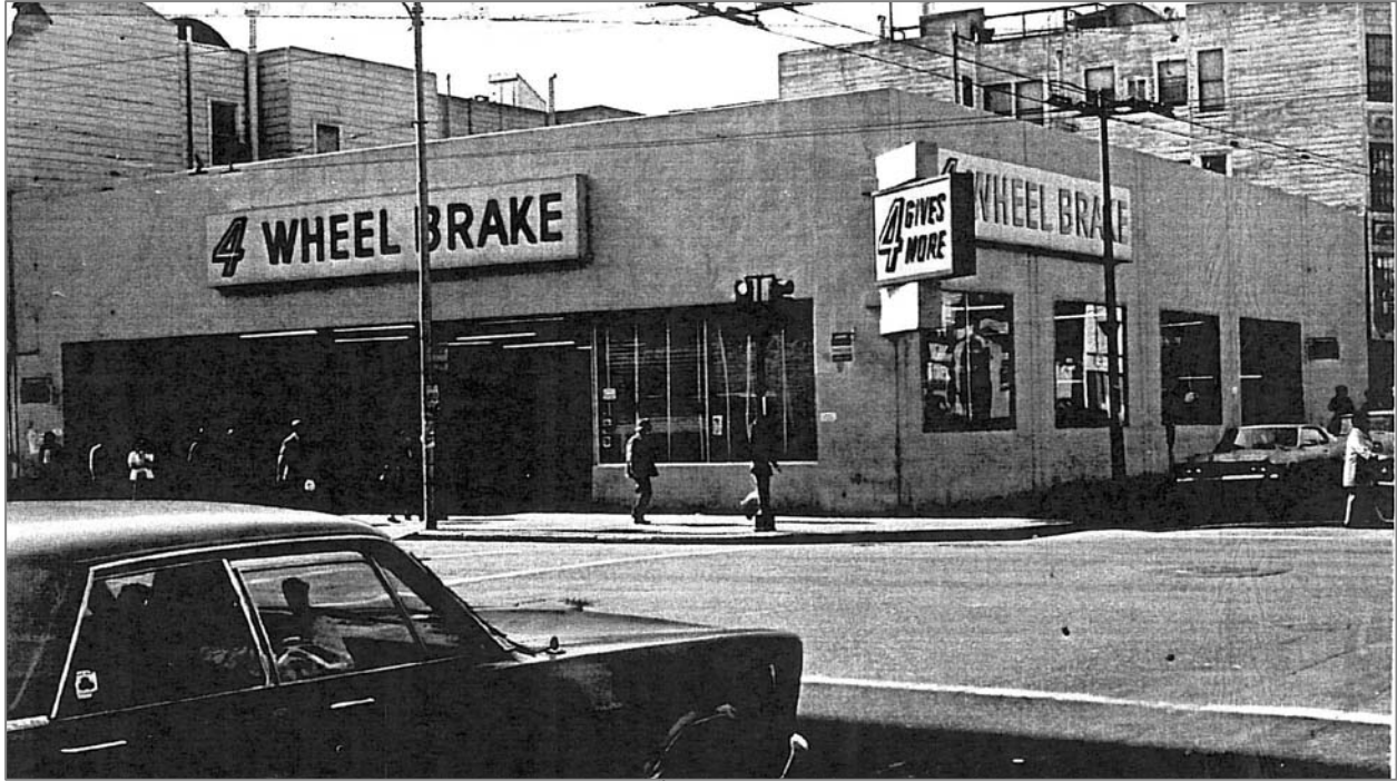
Figure 1 – Historic view from intersection of 17 th Street and Mission Street looking southwest. Image courtesy of San Francisco Office of the Assessor Recorder, building card, circa 1966.
