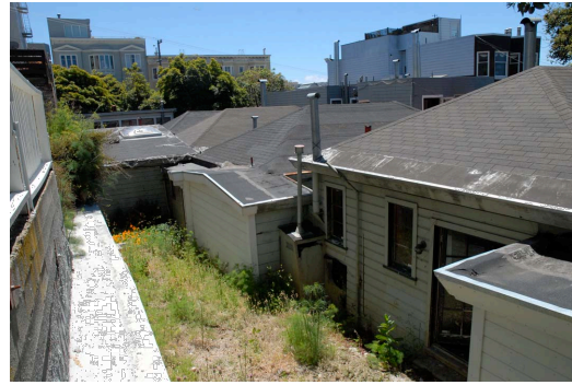
NON-CONTRIBUTING ADDITIONS @ COTTAGES B, C + D
