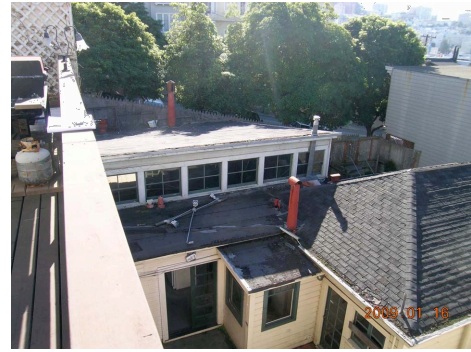
ROOF BETWEEN COTTAGE A + STUDIO
