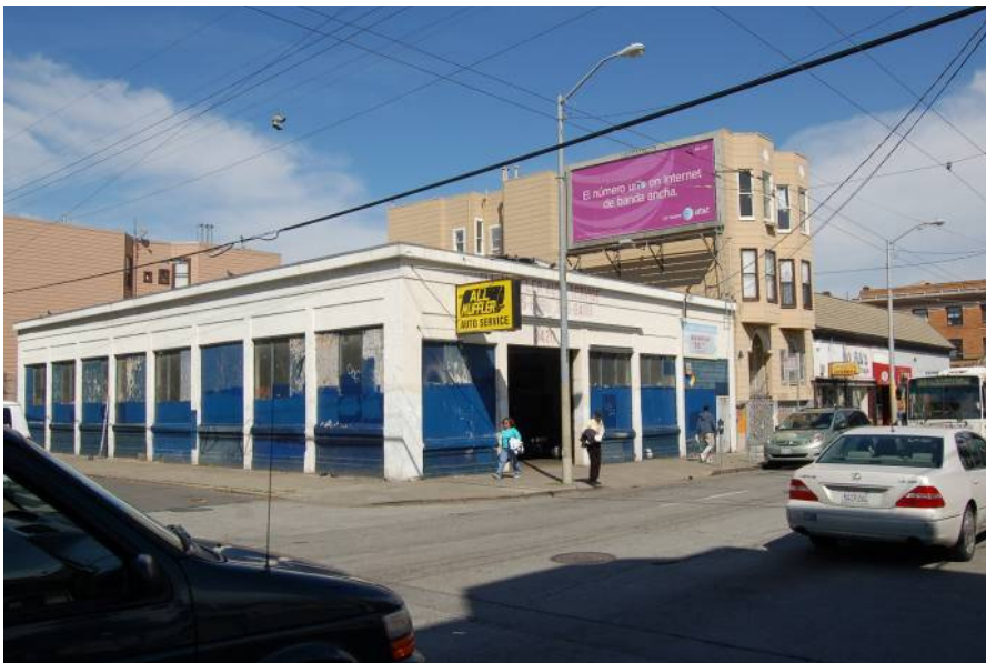
Photograph 2 3420 18 th Street, single story, simple cornice.
