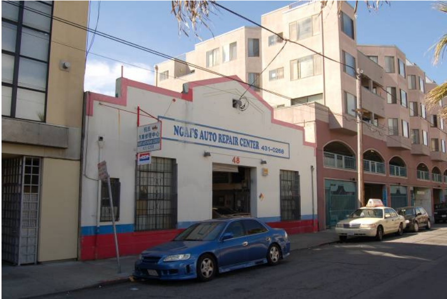
Photograph 5 48-50 Hoff Street, single story, parapet masks the roof profile.
