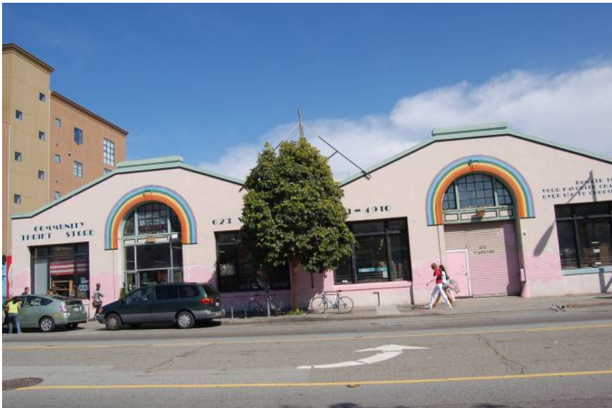
Photograph 4 623 Valencia Street, tapered parapet masks roof form. Like 25-35 Dolores, this property presents the appearance of paired buildings.
