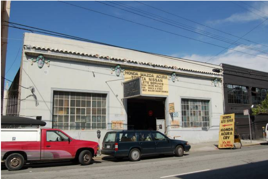
Photograph 1 280 14 th Street, Central door and cornice with tile and ornamental shields.
