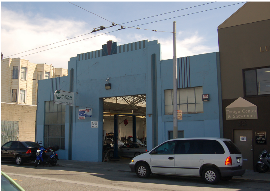
Photograph 6 3122 17 th Street, one story, trussed roof, Art Deco central door.
