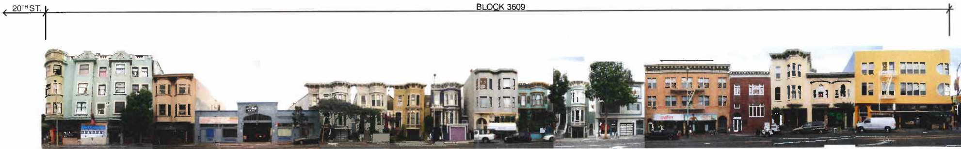
VALENCIA STREET: EAST SIDE
