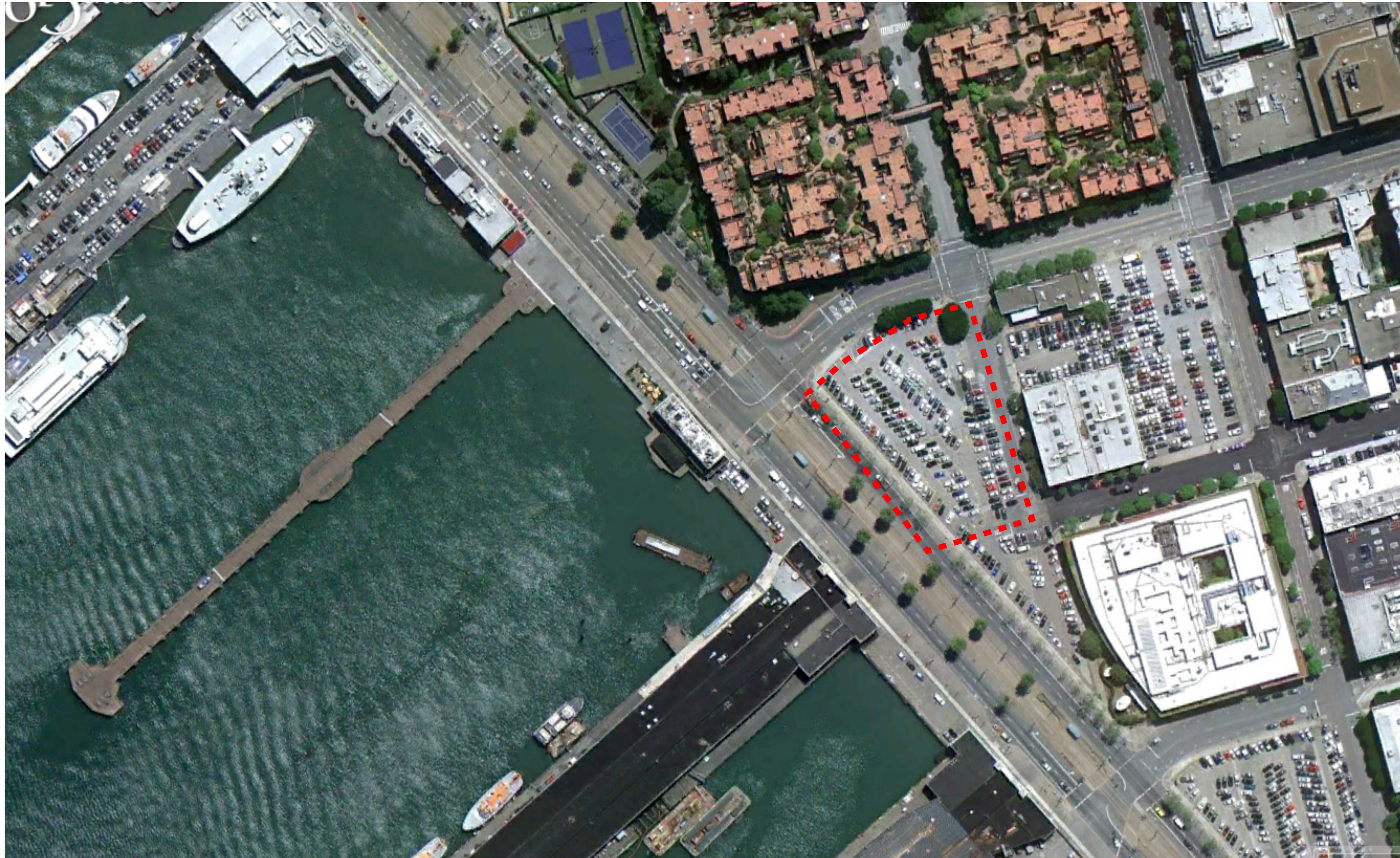
Current Surface Parking Lot
