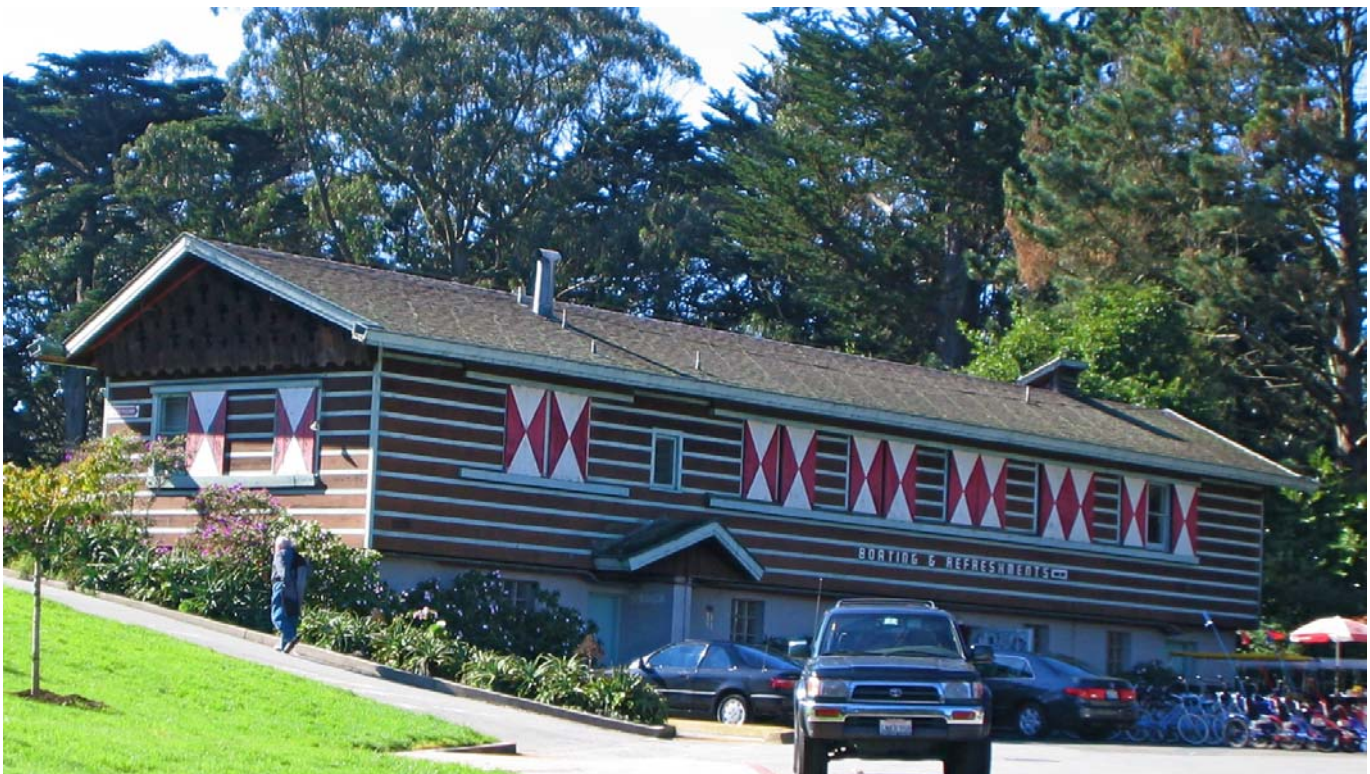
Current view of The Stow Lake Boathouse from parking lot.
