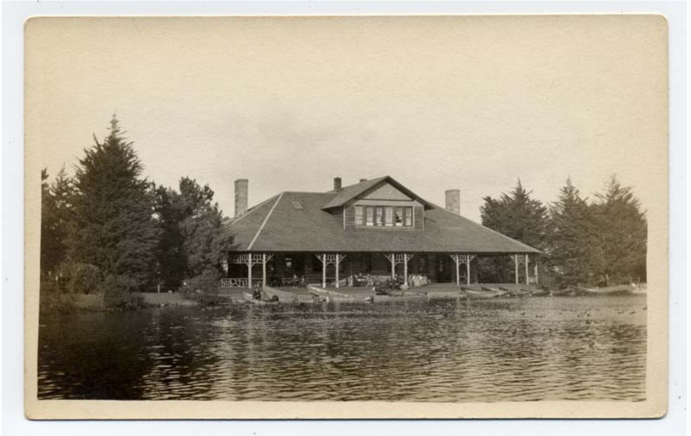
Photographic postcard view of the original boathouse lost to fire in the 1930's.
