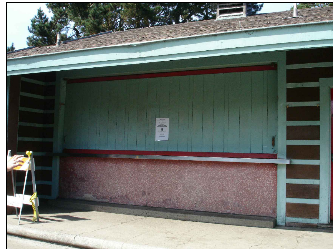
7 CONCESSION WINDOW—EXTERIOR A901
