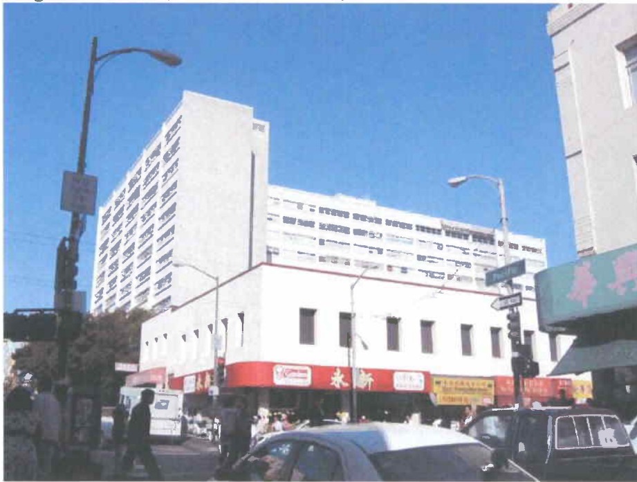
Looking west on Pacific Avenue
