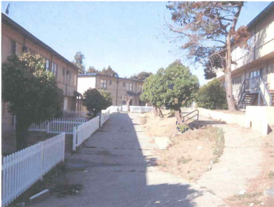
Looking into interior courtyards from Oakdale Avenue
