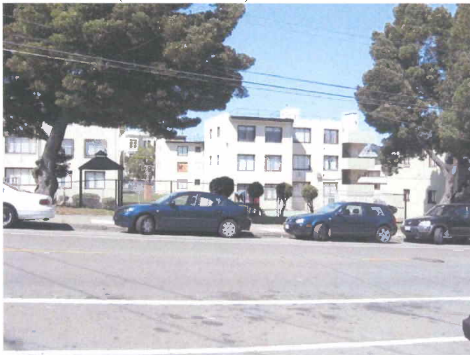
Looking north across Post Street
