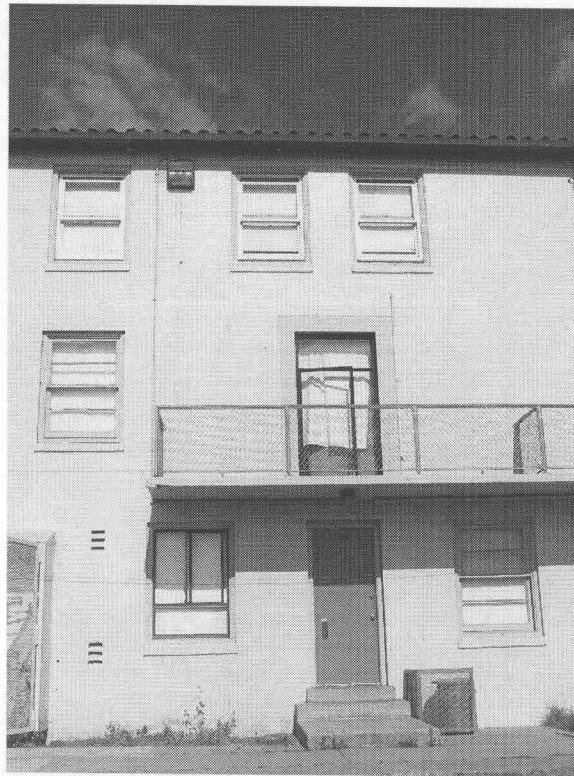
Photo 5: Detail of Front Elevation with Balcony
