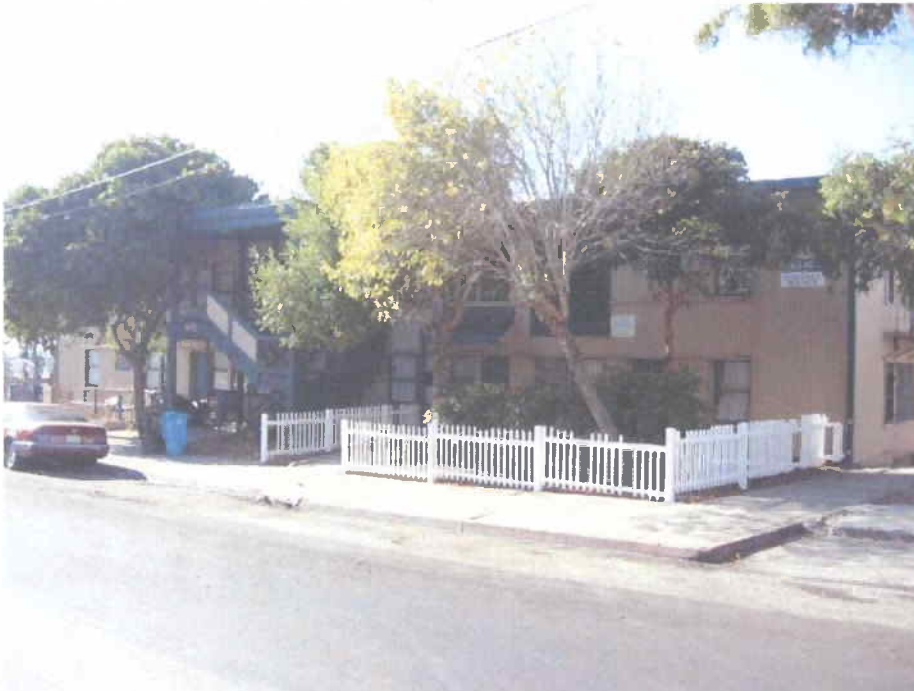
Primary elevation, building on Oakdale Avenue
