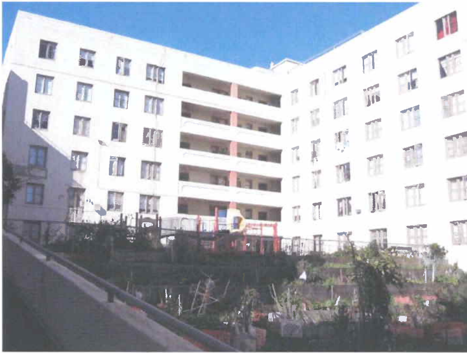
895 Pacific Avenue (rear courtyard/garden area)
