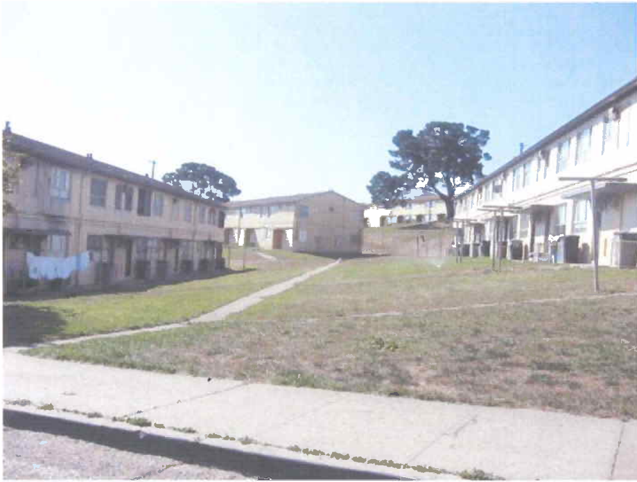
Concrete walkways and common space
