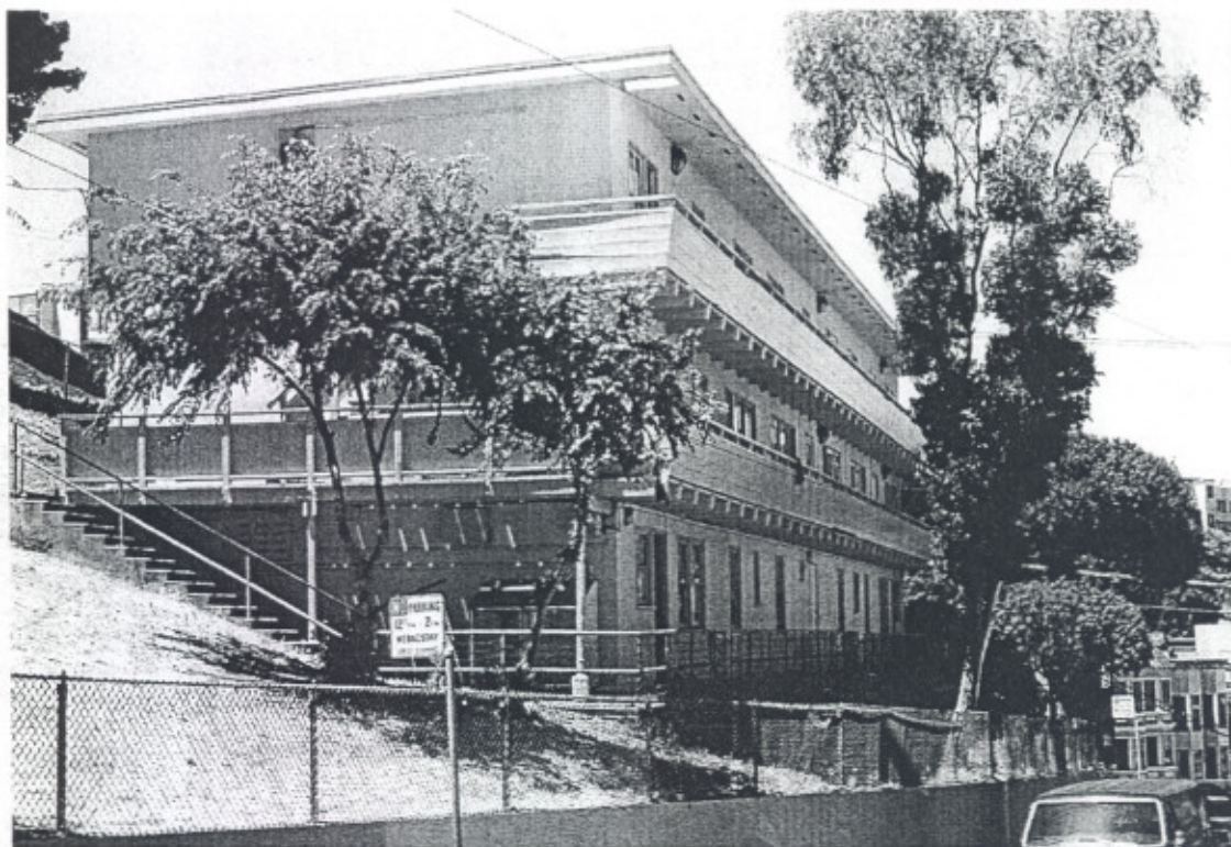
Photo 6: Side and Rear Elevation
