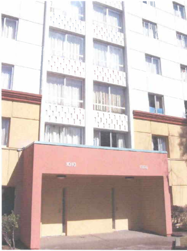
Secondary entrance along Webster Street
