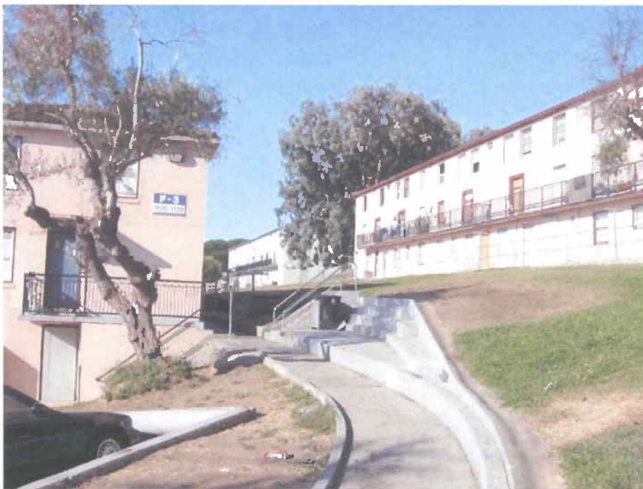
Concrete steps and walkways
