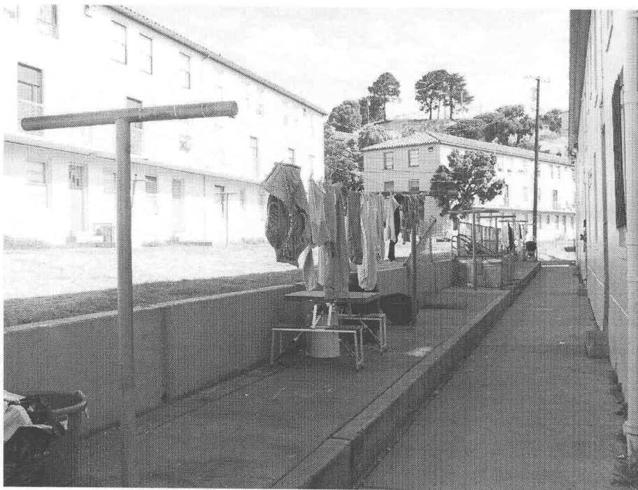
Photo 6: Laundry Area at Rear of Building
