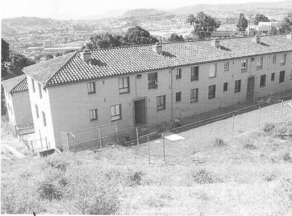
Photo 1: Rear Elevation of Building, View South
