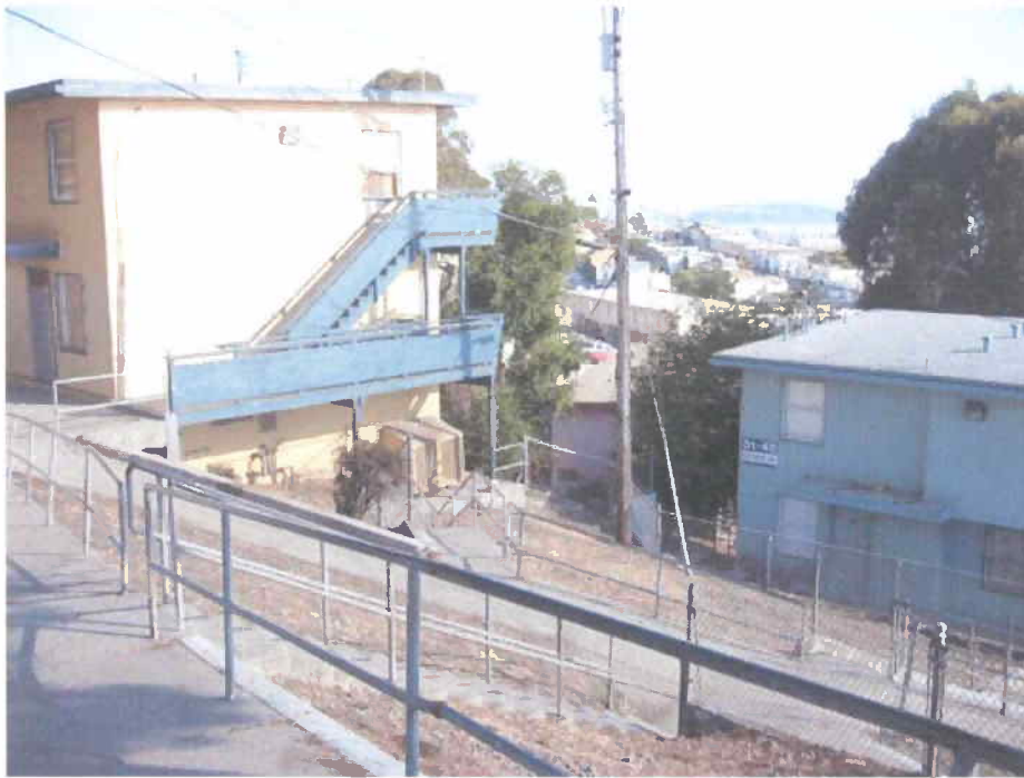
Concrete walkways and steps
