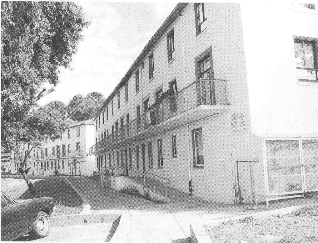
Photo 2: Front Elevation of Two Buildings, View North
