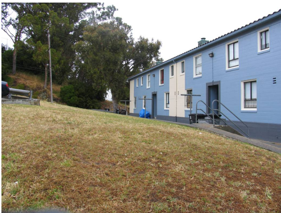
Fig. 7. This photo shows the typical landscaping behind a building. While these were generally open spaces, hedges often lined them and trees were planted close to the buildings. Note that virtually no formal plantings remain. Photo by Carey & Co., May 31, 2011.
