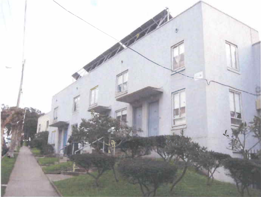
Looking west up Highland Avenue
