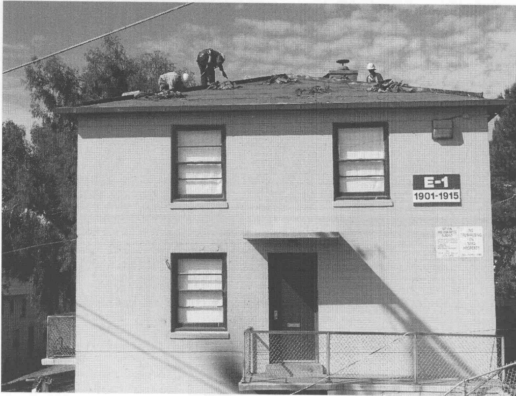
Photo 3: Side Elevation with Original Windows
