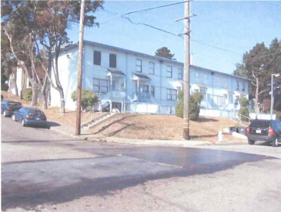
Front elevation, building at corner of Jerrold Avenue and Earl Streets
