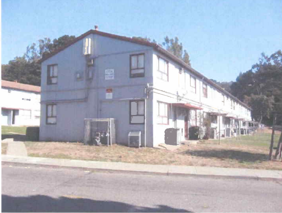
Two-story building along Sunnydale Avenue, primary elevation
