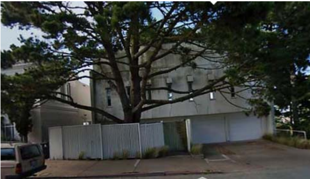
2009, 2010 photos Top: Side elevations Above: Street elevation
