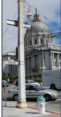
Van Ness trolley pole with single pendant and high pressure auxiliary water supply hydrant
