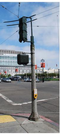
Modified aggregate concrete post with traffic signal
