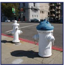
Low pressure fire hydrant and high pressure auxiliary water supply hydrant at Grove St
