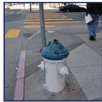
High pressure auxiliary water supply hydrant along Polk St
