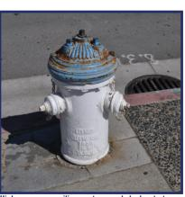
High pressure auxiliary water supply hydrant at Larkin St
