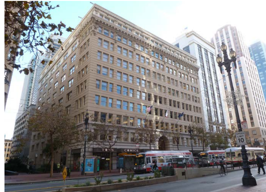
1 View along Market Street, looking southwest
