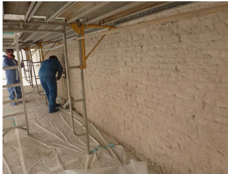
Annex wall after paint removal
