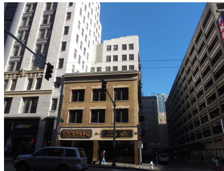
3 View from Third Street: Annex wall not visible
