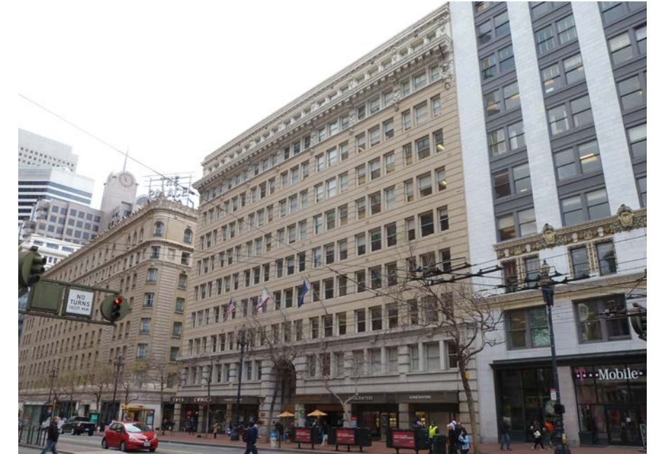
4 View along Market Street, looking east
