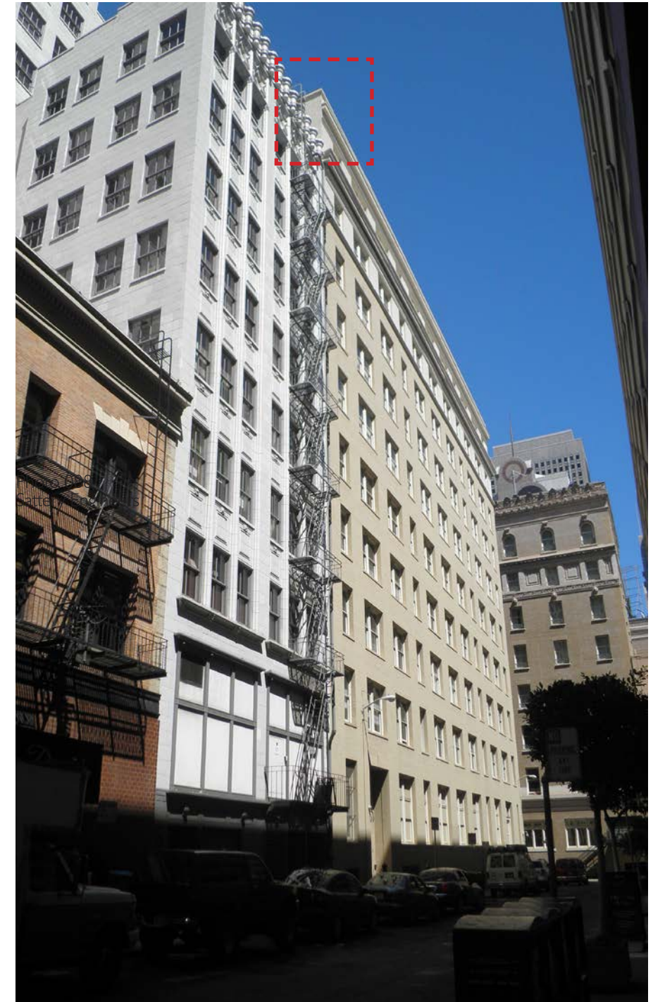
Stevenson Street Facade (Annex wall shown in dashed rectangle)
