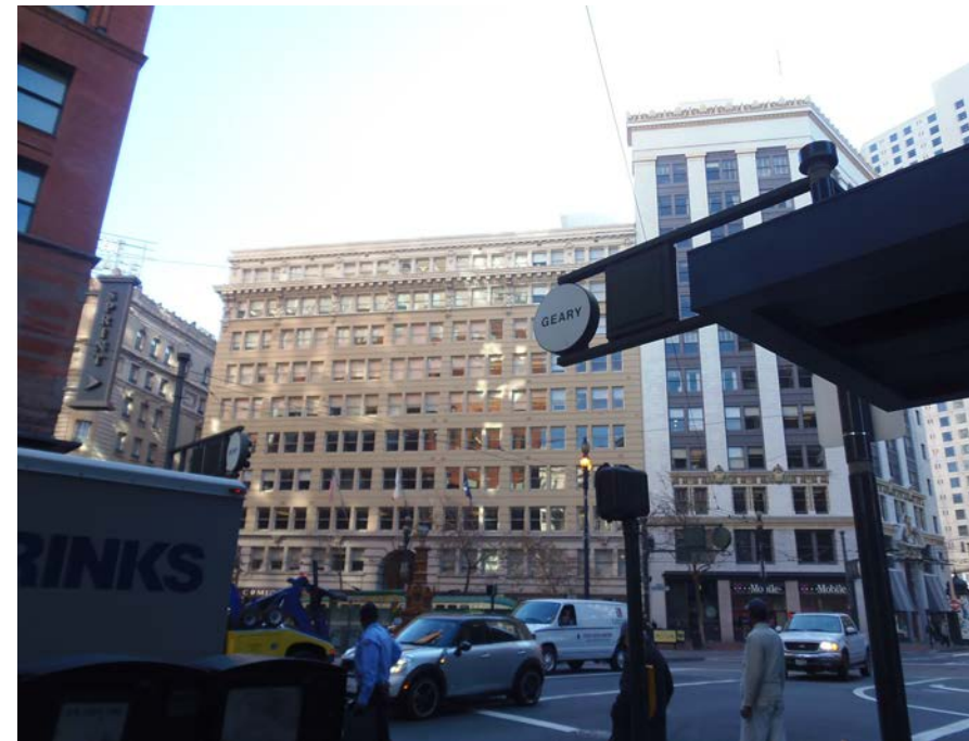
1 View from Market Street: Annex wall not visible
