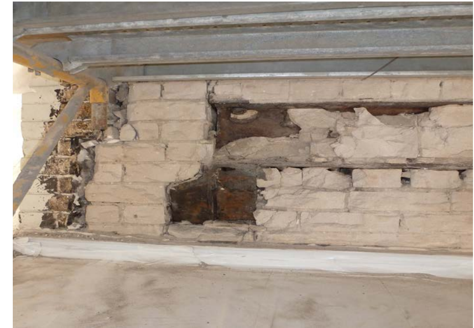
Photo of deteriorated brick at Annex wall
