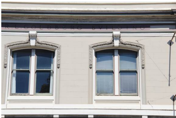
R. L. Goldberg Building, 182-198 Gough Street
