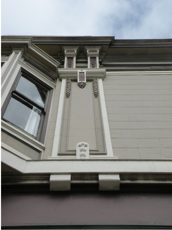
Figure 3 Classical elements from the Beaux Arts palette including the measured use of moldings to create crisp cornice and panel elements create an impression of exceptional refinement and design quality to R. L. Goldberg Building's edifice.
