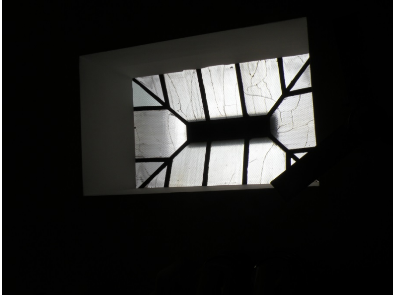
Figure 43 Looking up at the hip-form skylight in the center of the ceiling of 190 Gough Street. The skylight is set at the foot of the central lightwell.
