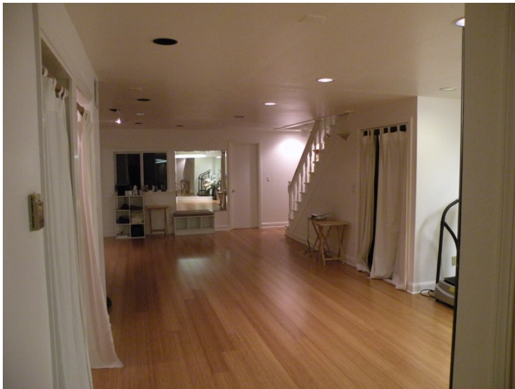
Figure 44 The basement of the central commercial unit, 190 Gough Street, has been finished in drywall. Original stair balustrade and wood door surrounds were left in place.
