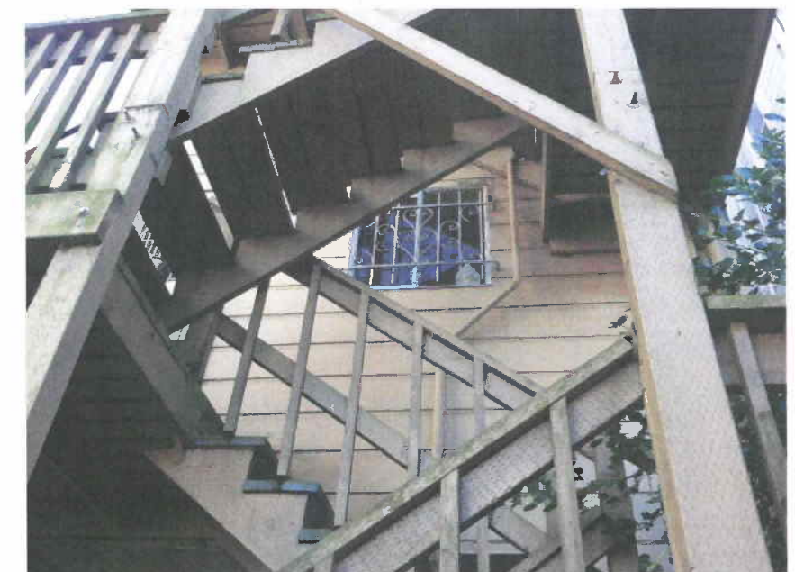
EXISTING REAR STAIR
