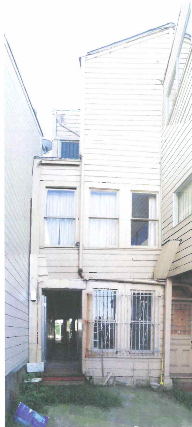
EXISTING NORTH FACADE FROM REAR YARD
