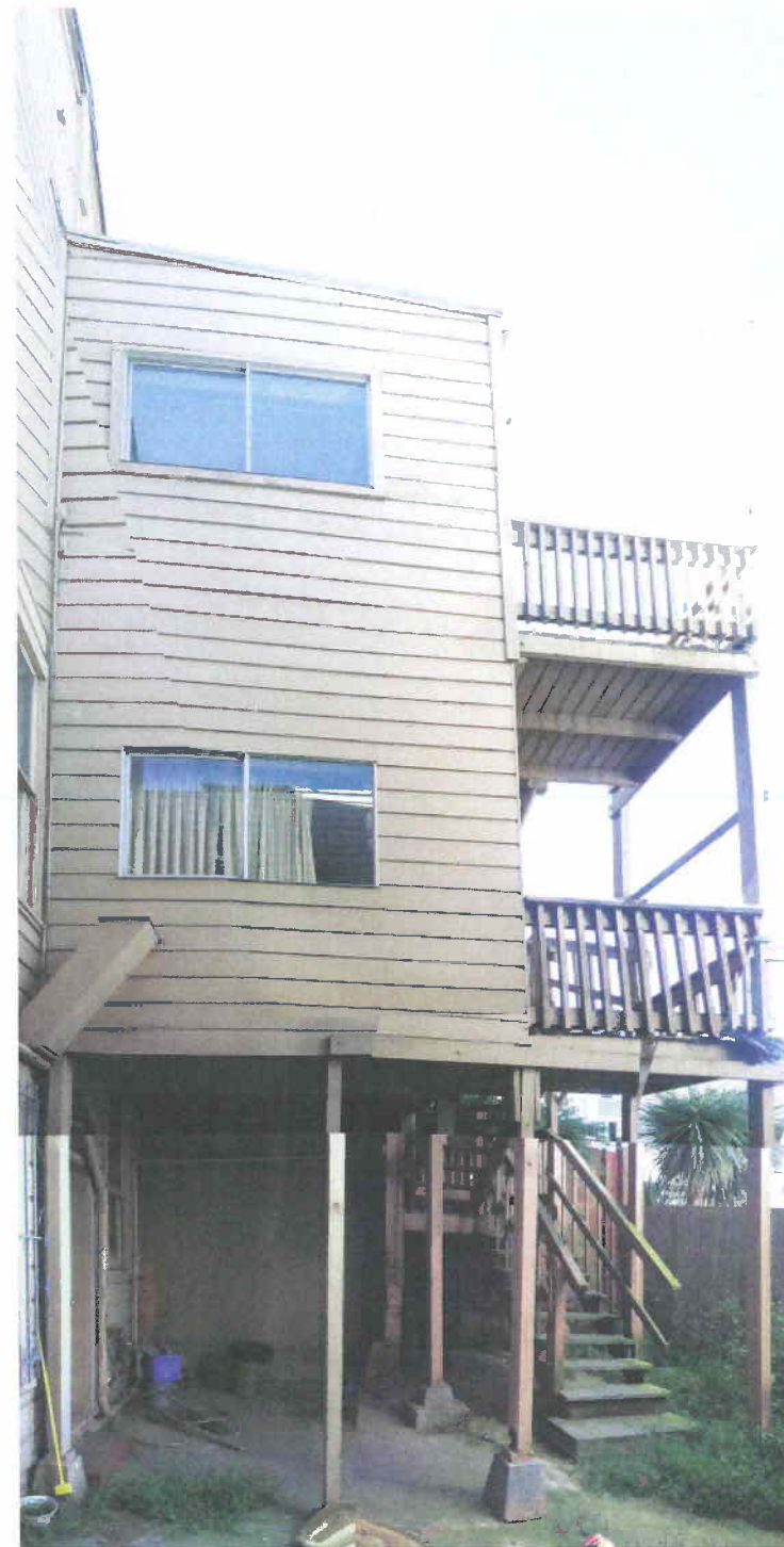
EXISTING EAST FACADE FROM REAR YARD
