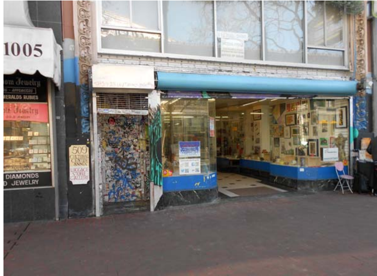
Figure 24. Ground floor with doorway and storefront. [No. 1322] January 2014
