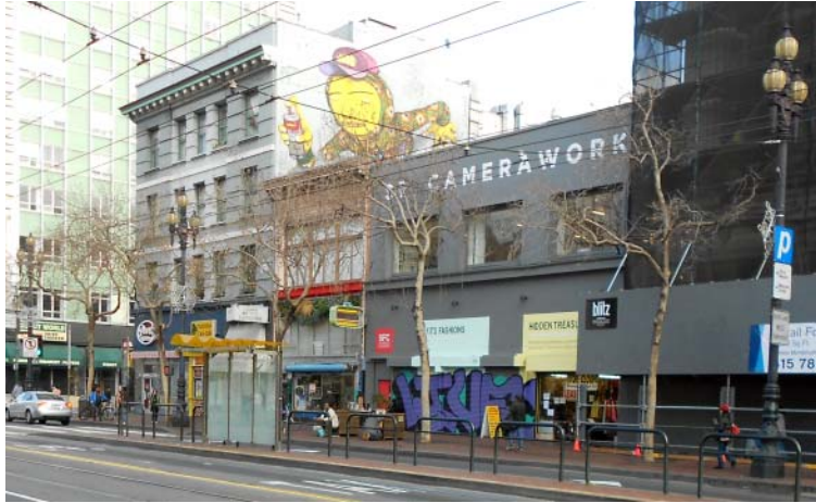
Figure 1. View east showing the Walker Building in its context on the south side of Market Street. [No. 15.54.33] January 2014.
