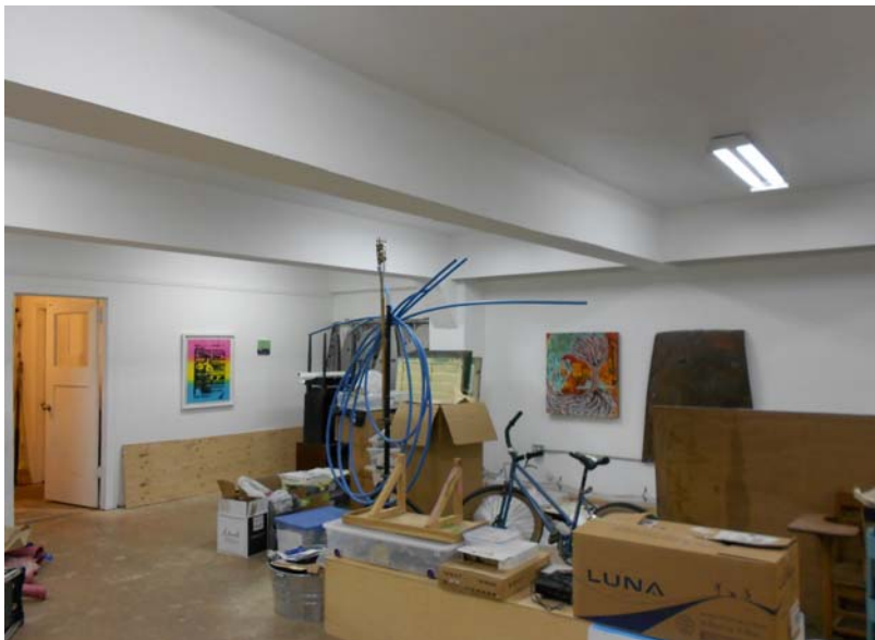
Figure 19. Interior view south on mezzanine floor showing concrete clad steel post-and-beam construction. [No. 16.25.40] January 2014.
