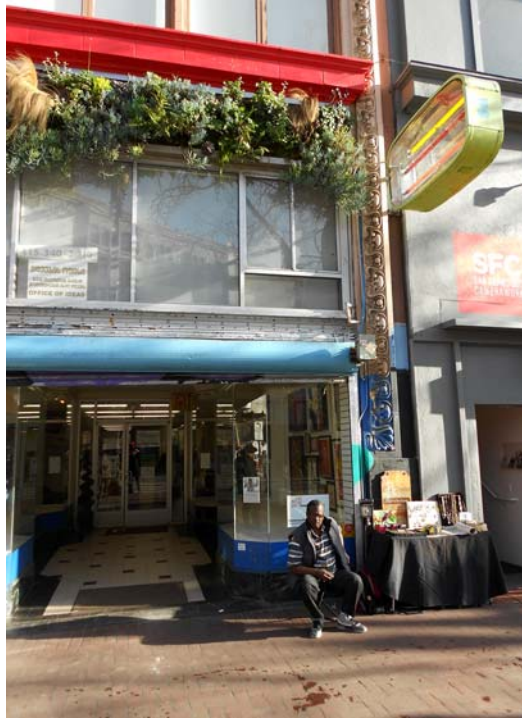
Figure 7. Storefront detail including cantilevered sign added to west pier 1970s-1980s. [No. 17.22.47] February 2014
