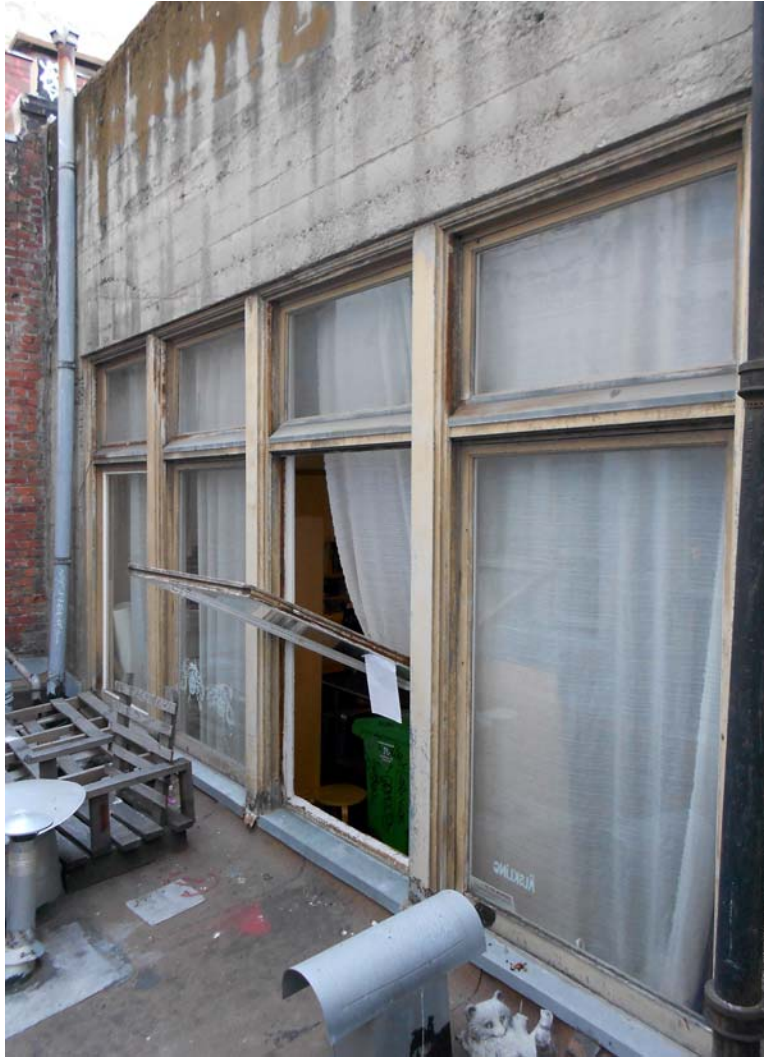
Figure 20. View west showing rear wall of second floor. [No. 16.57.37] January 2014.
