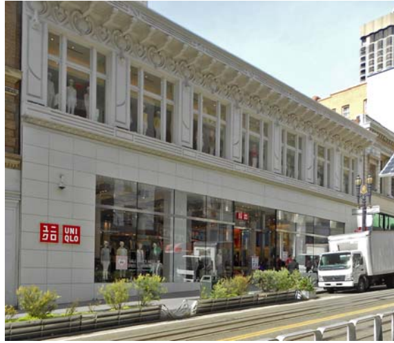
Figure 35. 133 Powell Street. View north. [No. 13.30.20] February 2014.
