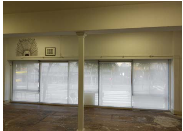
Figure 11. Interior view northwest on mezzanine floor toward windows facing Market Street. [No. 16.25.16] January 2014.
