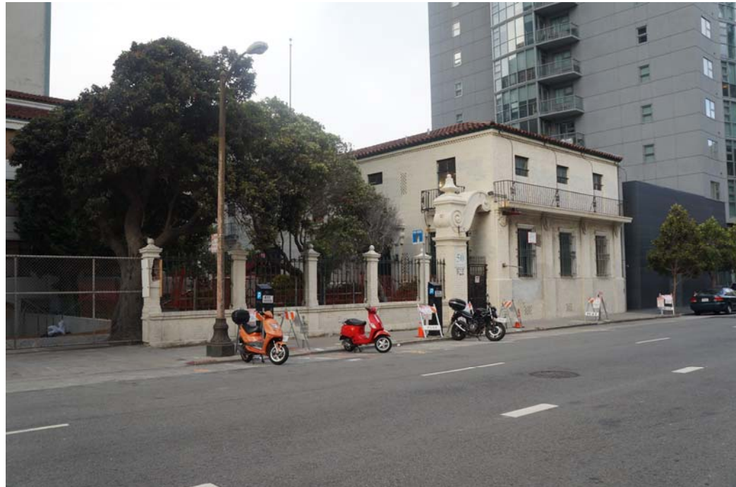
View looking northeast from across Fell Street at the site wall and East Wing (Knapp, 2014).
