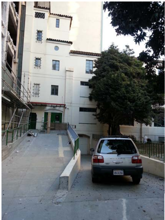
Image 2 – View from Fell Street to north wing tower, non-historic ramps and drives in the foreground. (Knapp, 2013)
