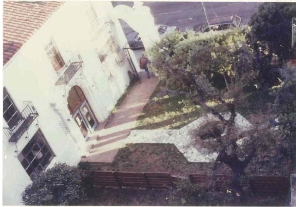
View of courtyard from upper story of North Wing with historic fountain base at center. (Planning Department Files, Date Unknown)
