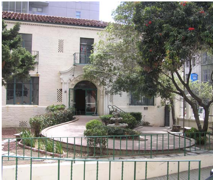
Image 3 – East wing looking east with non-historic curvilinear ramp in foreground. (Knapp, 2013)
