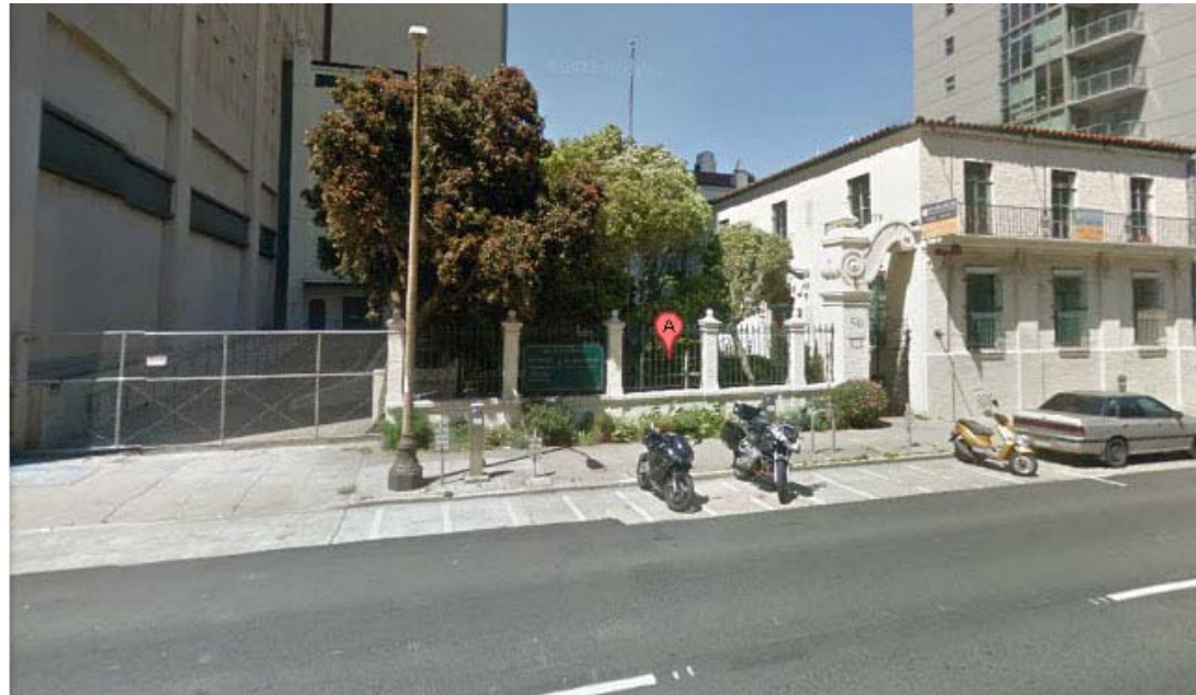
Image 6 – View along Fell Street looking northeast, east wing at right. The west side of the yard wall is missing. (Google, May 2011)
