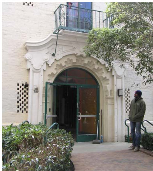
Image 8 – View of decorative arched entry at east wing looking east. The lower portion of original pilasters has been covered where the non-historic brick ramp and concrete steps were installed and interior steps were infilled with new floor to meet the ramp landing. (Knapp, 2013)
