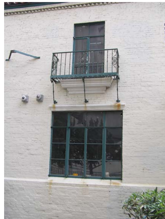
Existing Areas of Major Permit to Alter Scope: Top: (5) Non-historic retaining wall removal; Bottom: (6) New exit doors at existing first floor window openings near the corner of the L-shaped building at the North and East Wings. The existing historic window at each location will be salvaged and stored. The new door with sidelights will be detailed similarly to the existing windows.
