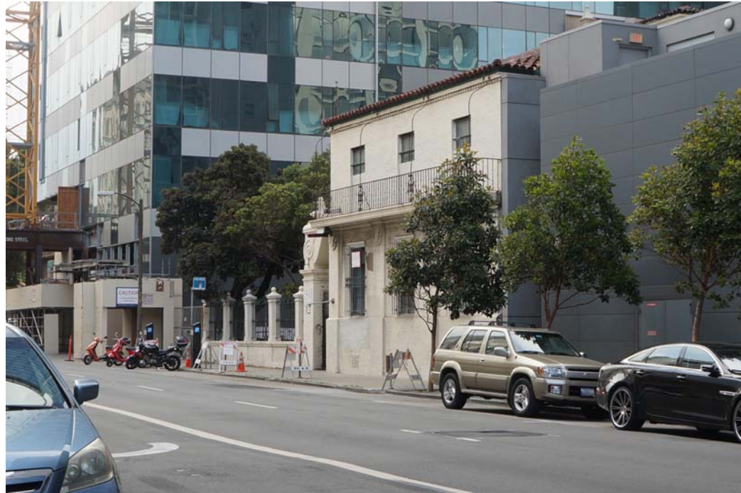
View looking northwest from across Fell Street at the East Wing and site wall (Knapp, 2014).
