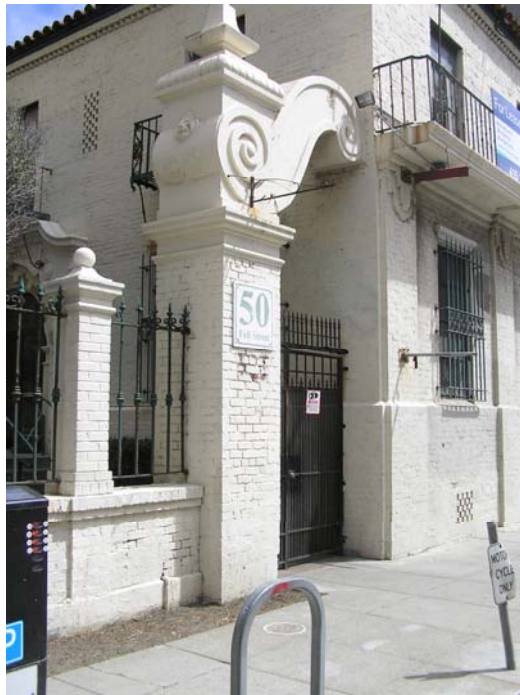
Image 7 – View of decorative arched gateway with non-historic gate looking northeast from Fell Street. (Knapp, 2013)
