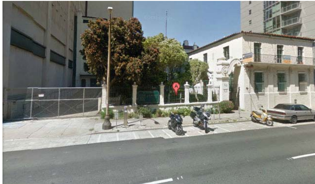
Image 6 – View along Fell Street looking northeast, east wing at right. The west side of the yard wall is missing. (Google, May 2011)
