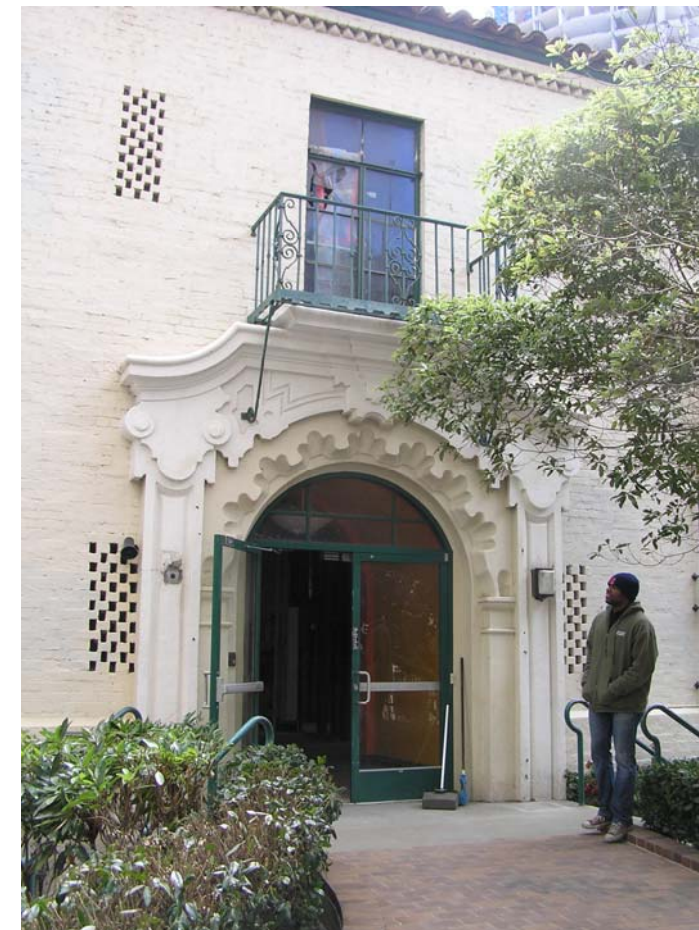
Main East Wing Entry
