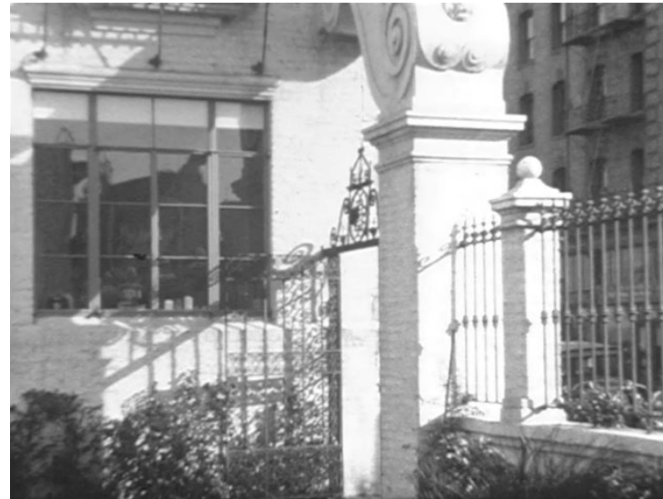
Image 7A – Historic view of decorative arched gateway with original wrought iron gate at yard wall looking southeast from the yard. (Viavi Brand Products Archives. Film, circa 1931. Images cannot be publically posted or reproduced without permission from Wayne Vico / Viavi)
