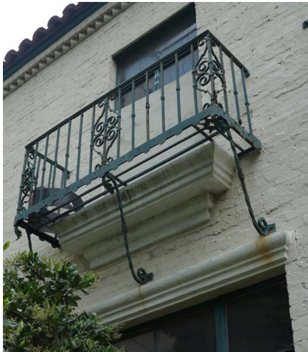
Existing Areas of Major Permit to Alter Scope: Top row –(1) Historic site wall reconstruction at west end, (2) Historic wrought iron (A36 Steel) fence reconstruction; Bottom Row – (3) Historic wrought iron (A36 steel) balcony rehabilitation; (4) New west gate assembly to replace existing chain link gate.
