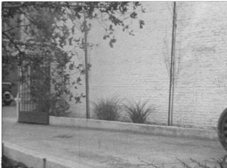
Image 2B – Historic view of driveway along west side of property looking southwest. (Viavi Brand Products Archives. Film, circa 1931. Images cannot be publically posted or reproduced without permission from Wayne Vico / Viavi)
