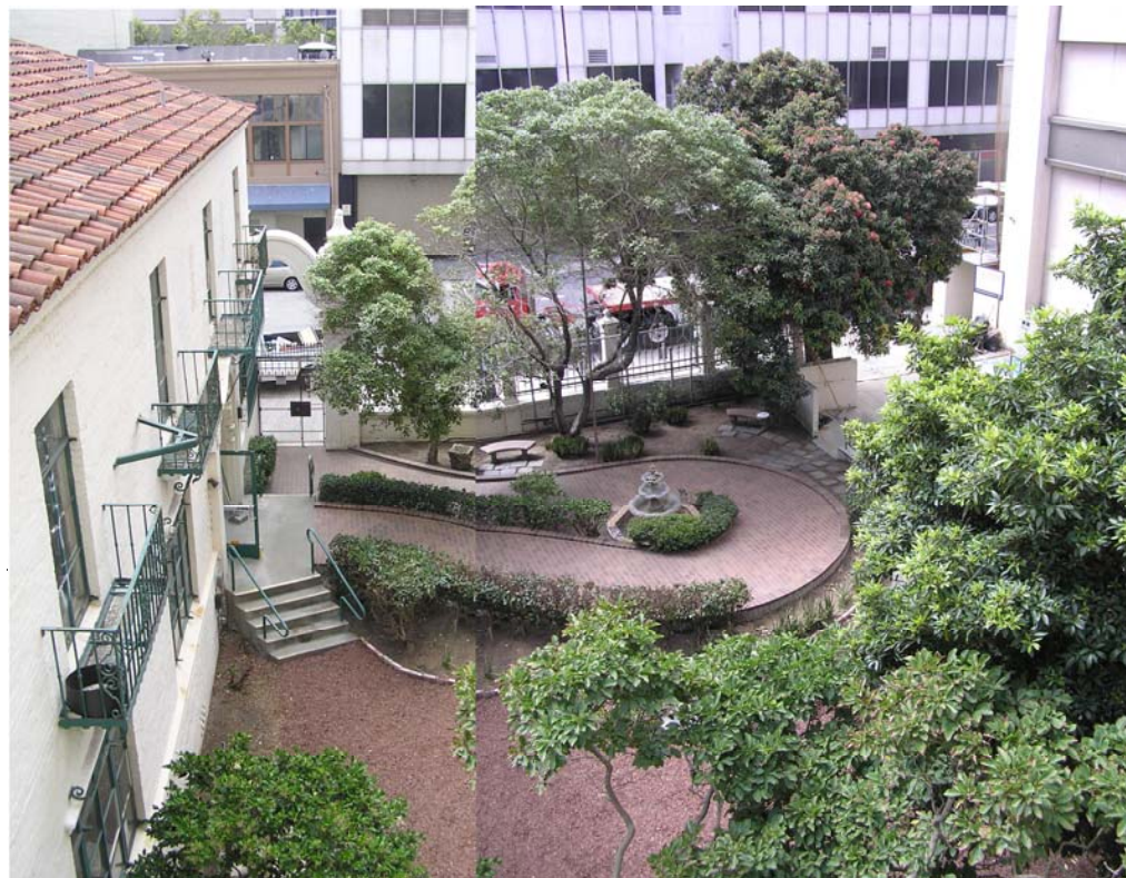
View of courtyard from upper story of North Wing with historic fountain base relocated within non-historic curvilinear brick ramp. (Knapp, 2013)
