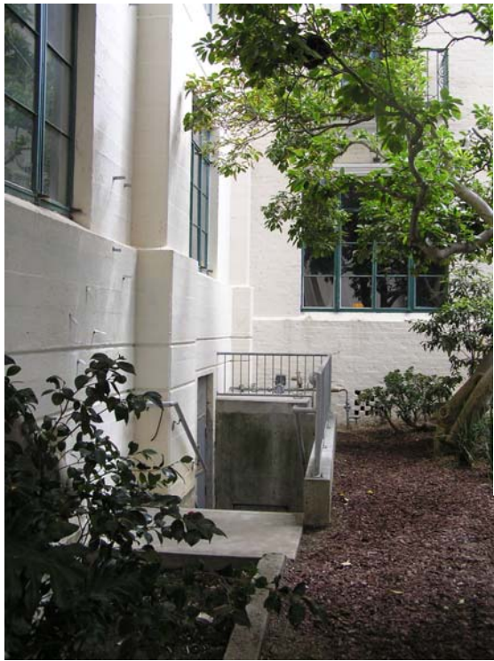
Image 1 – Non-historic basement stair at corner between east and north wing. Historic window modified to doorway to basement. (Knapp, 2013)
