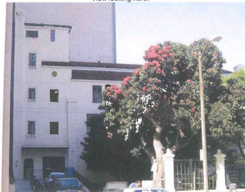
Service entrance and stair tower
