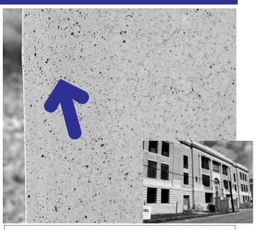
Where's the Repair? Glazed terra cotta spall, upper left corner, filled and smoothed using Thin-Fill 55 prior to glazing and speckling with Aquathane UA210 coatings, matched to original glaze colors. Project is an Historic school restoration in Charleston, SC.
