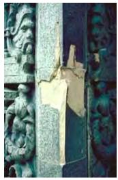
The damage shown here is the result of direct live load on a mid-rise building. The steel frame has settled and shifted the weight onto the exterior terra-cotta cladding, resulting in rupturing of the material. Photo: NPS files.
