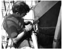
patches, cool and damp conditions). At temperatures below 50F (10 C), use of RL-6 winter grade latex is recommended to accelerate curing.
