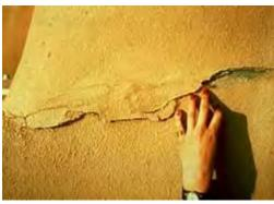
A waterproof coating is an inappropraite substitute material to apply to adobe as it seals in moisture and may result in spalling. Photo: NPS files.
