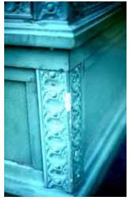
Substitute materials need to be located with care to avoid damage. The fiberglass column base has chipped, whereas the files.
