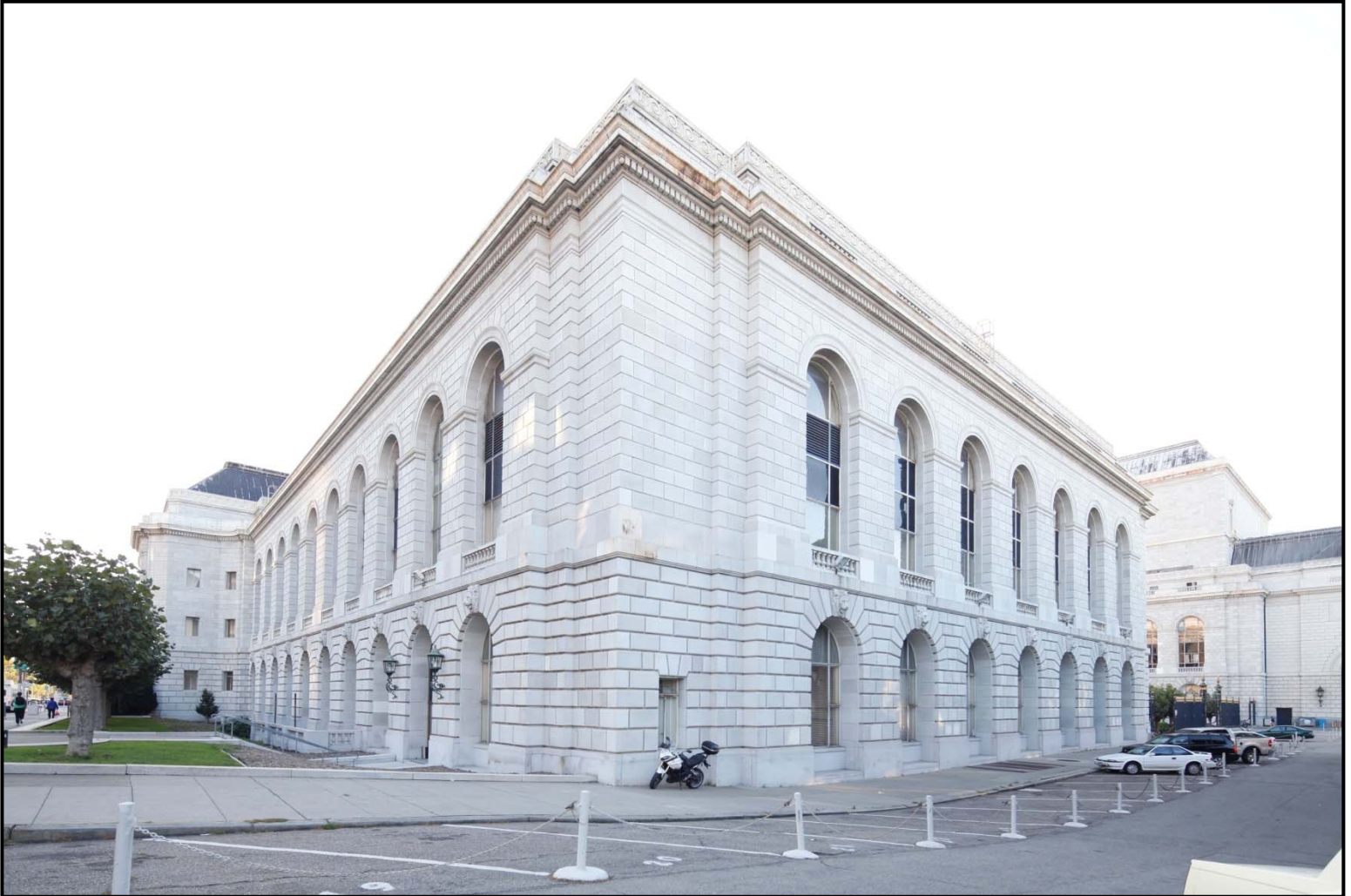
View of Veterans Building , North and West Facades
