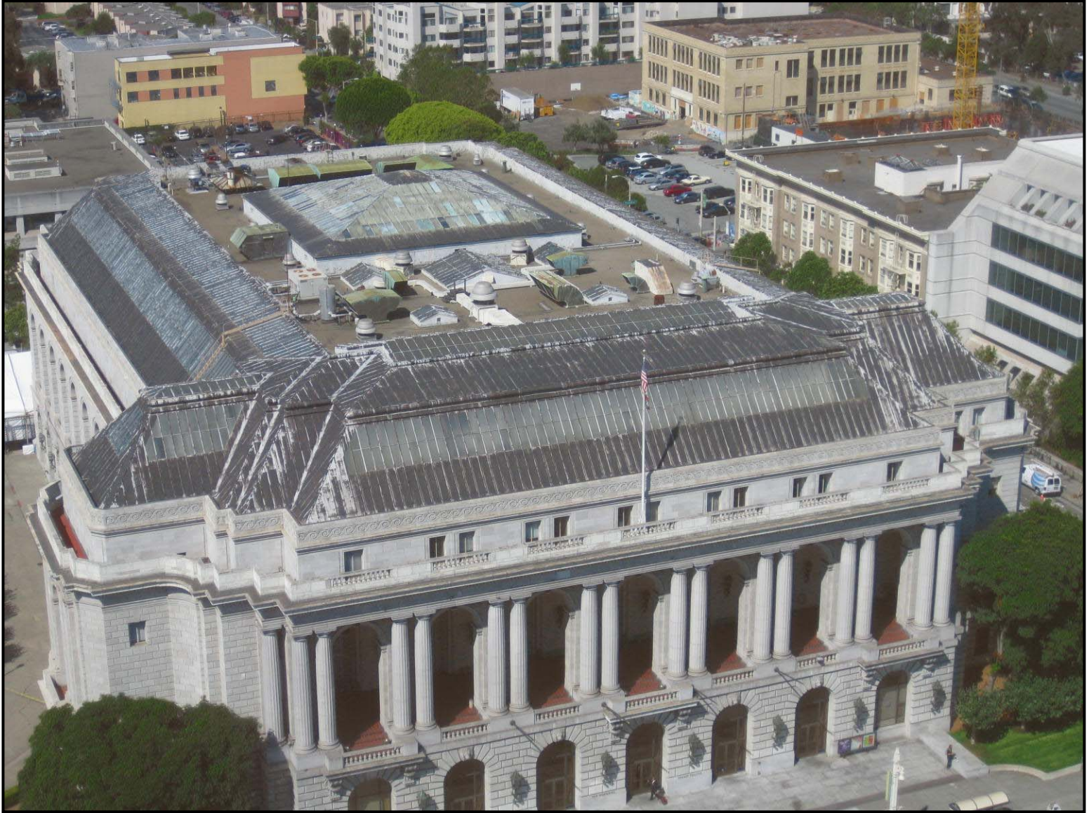
View of Veterans Building Roof
