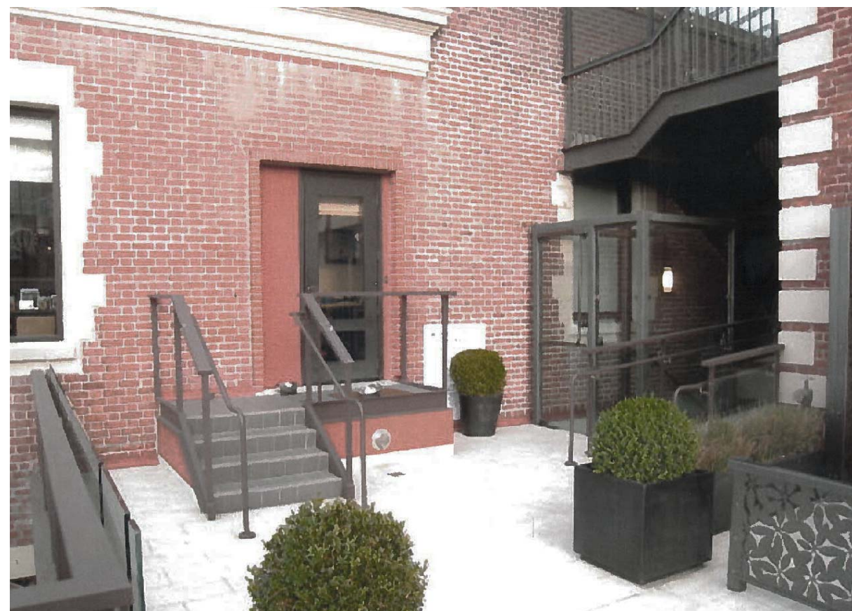
EXISTING STAIR PHOTOGRAPH
