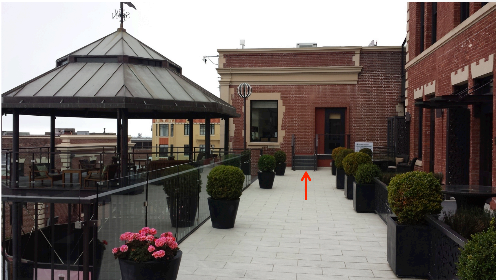
Existing landing looking East from private residence club's shared terrace
