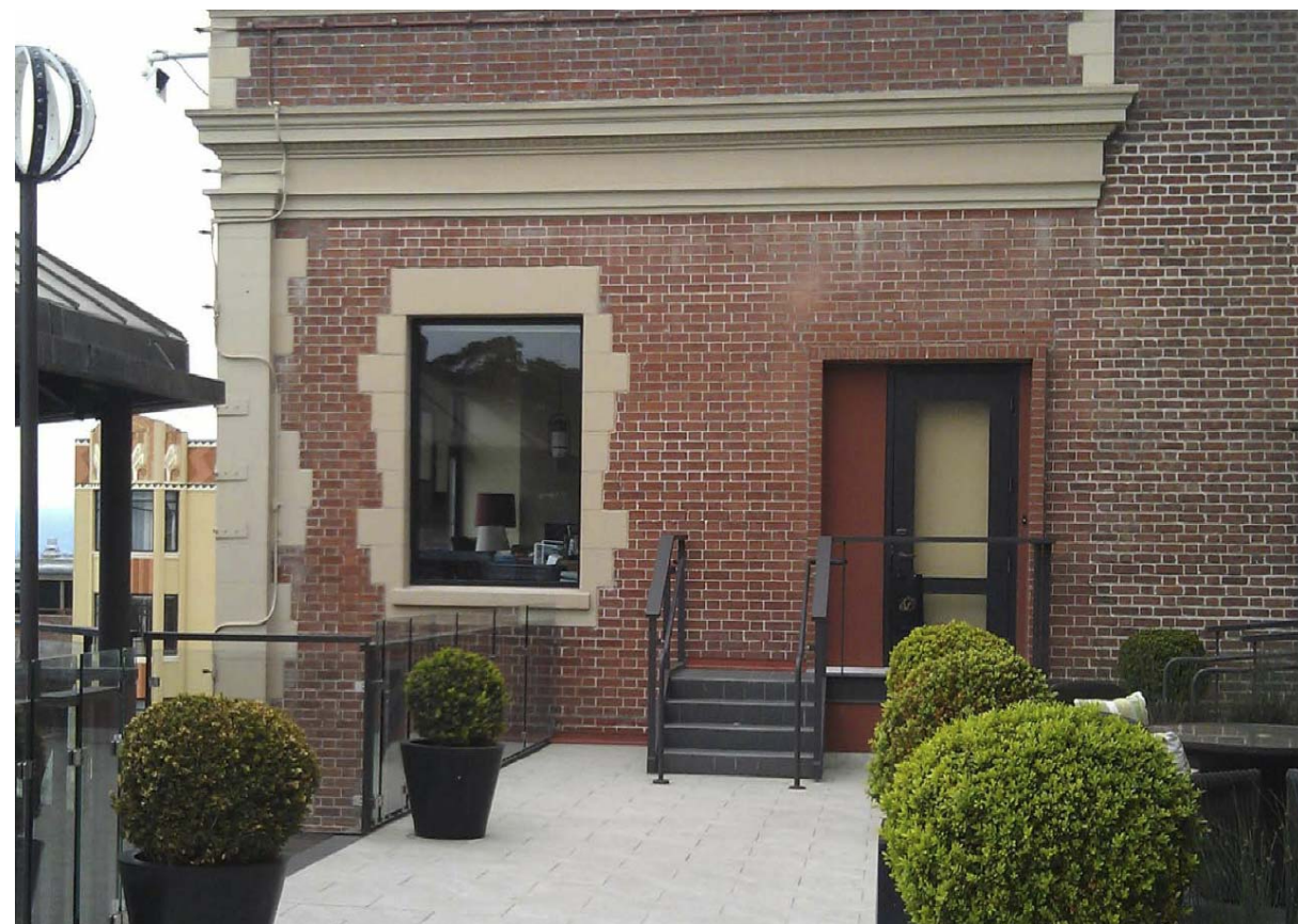
EXISTING STAIR PHOTOGRAPH
