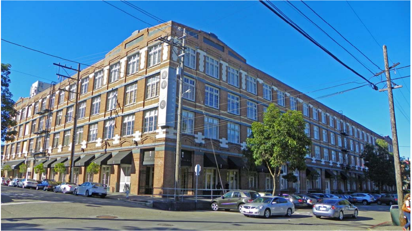
East facade (r), south facade (l)
