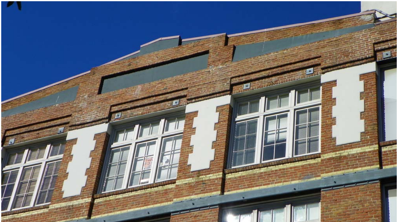
Detail: Peaked parapet and quoin-like panels (south facade)
