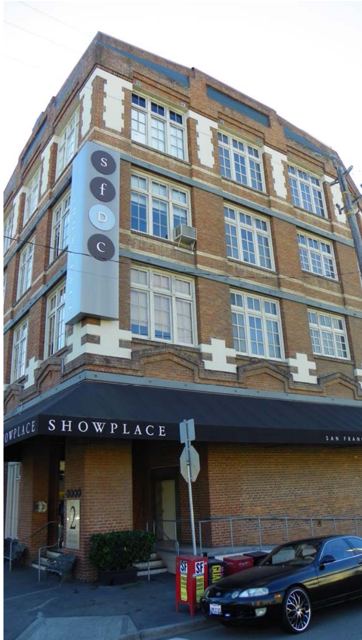
North facade (r) east facade (l)
