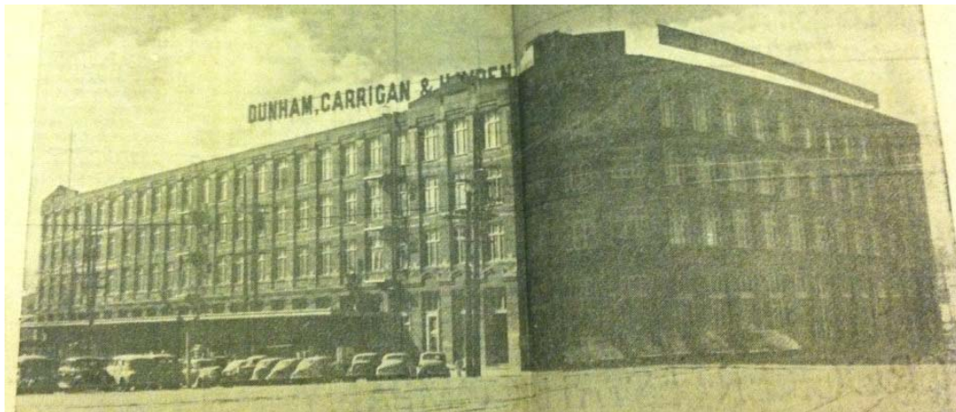
Dunham, Carrigan & Hayden Company building, 1948 ("100 Years in San Francisco," San Francisco Chronicle, 18 Oct 1948)
