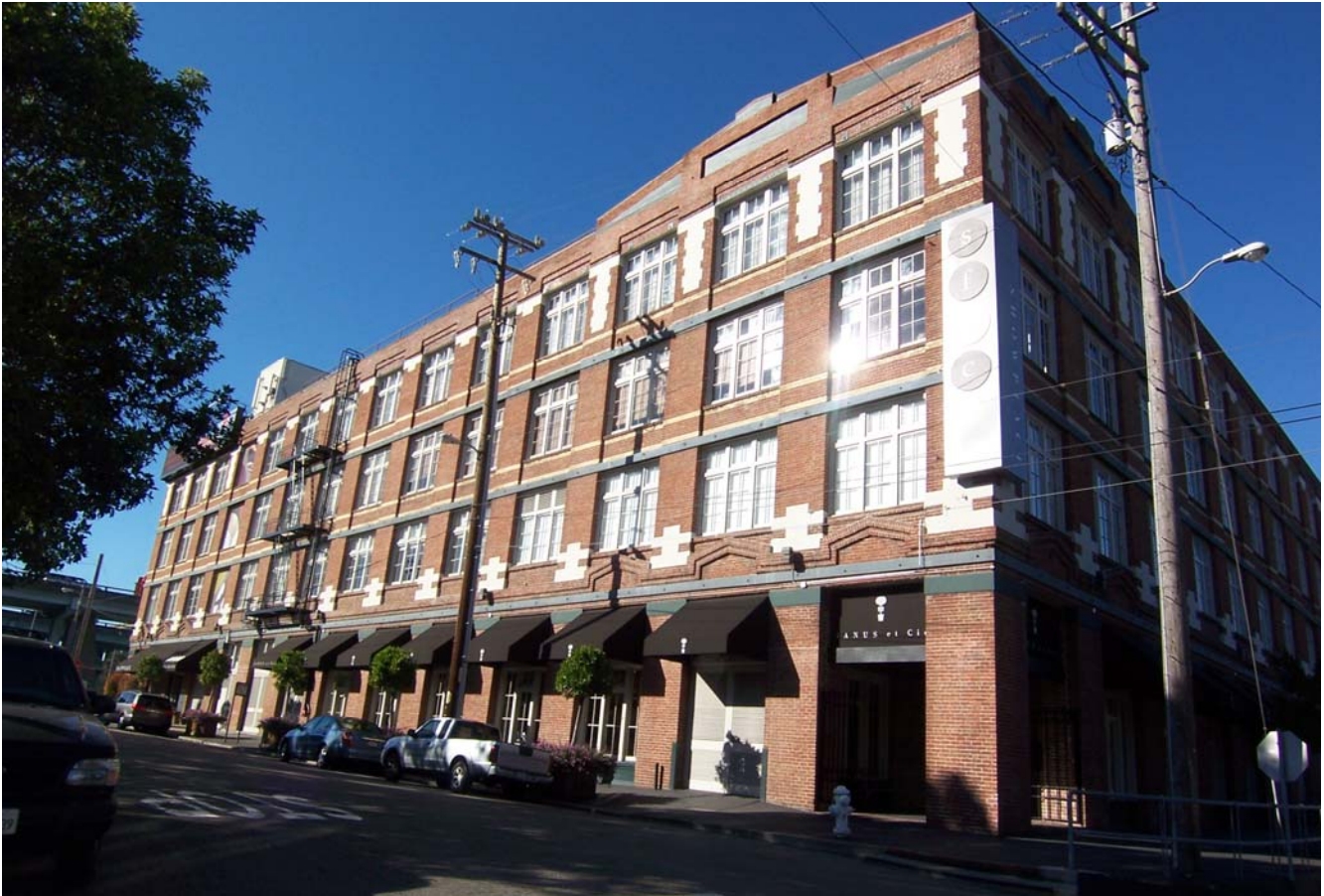
South facade (l), east facade (r)
