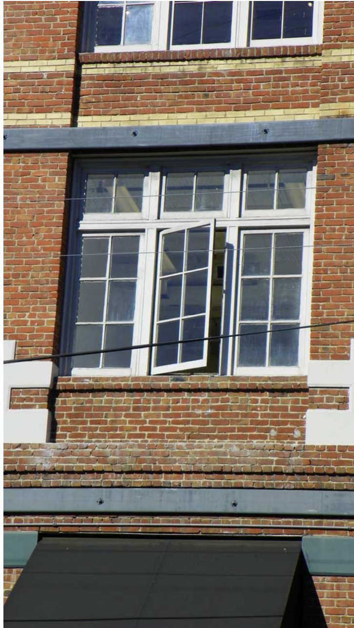
Typical upper story windows
