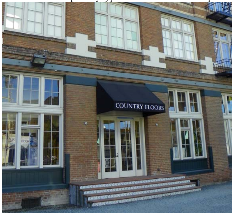
Detail: Contemporary exterior stair, northwest facade
