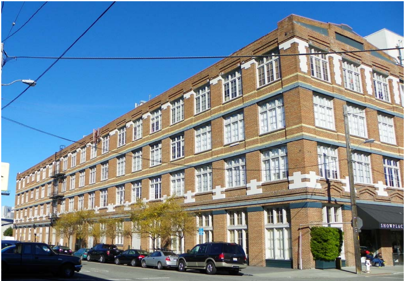
West facade (l), south facade (r)
