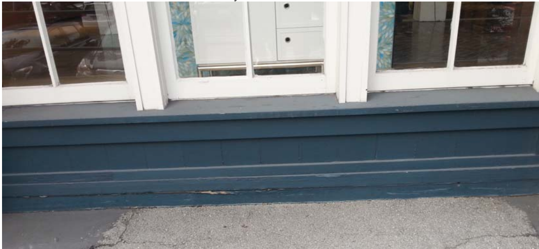
Solid wood bulkhead
