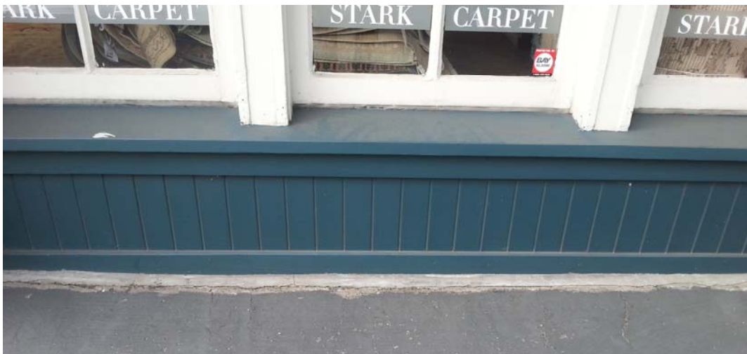
Vertical board bulkhead
