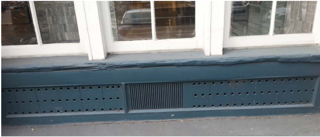
Perforated bulkhead
