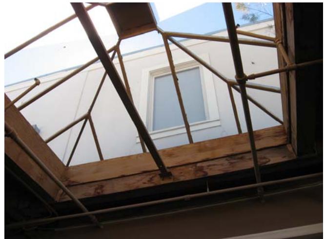
Example of skylight on fourth floor.
