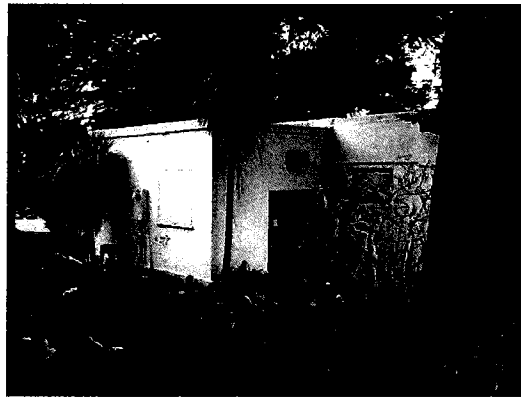
Figure 24. Rear façade of convenience station. Source: Page & Turnbull, January 2012.
