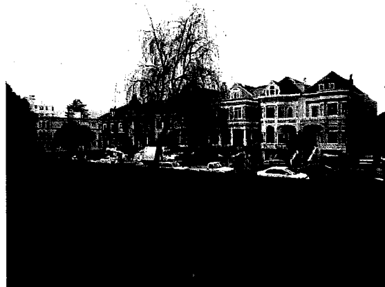
Figure 45. View southwest toward Scott Street, between Grove and Fulton streets.
