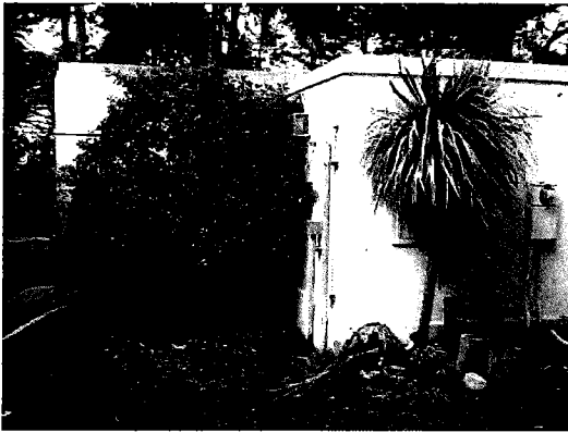
Figure 23. Rear façade of convenience station. Source: Page & Turnbull, January 2012.
