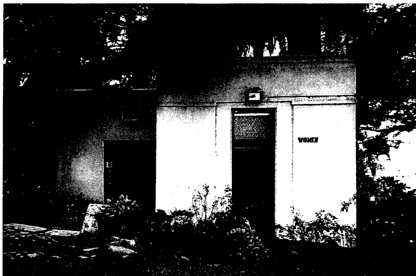
Figure 21. East façade of convenience station. Source: Page & Turnbull, January 2012.
