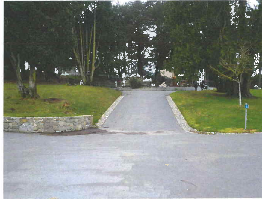
River rock gutters and a rock-faced wall, looking west toward playground.
