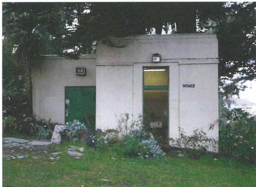
East façade of convenience station.
