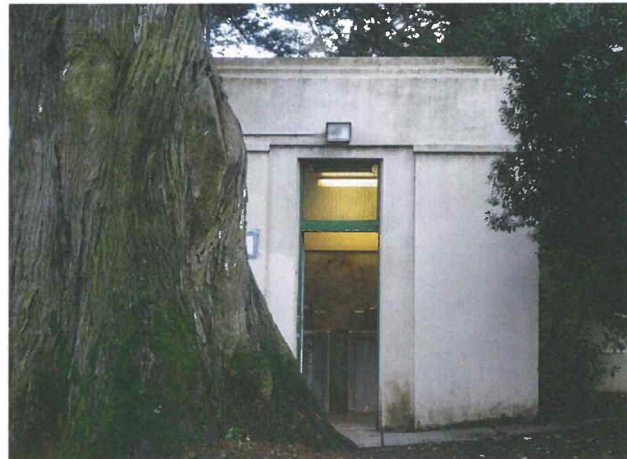
West façade of convenience station
