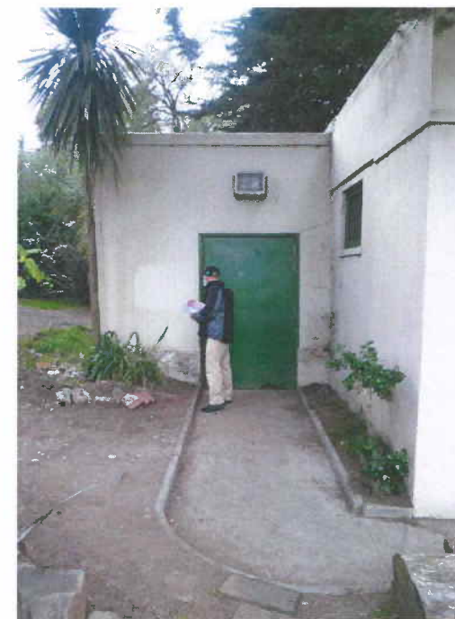
East facade entrance
