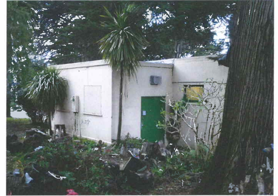
Rear façade of convenience station
