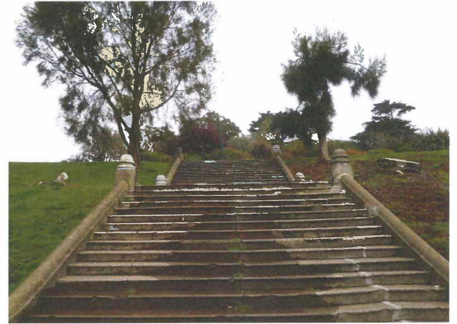
View of Scott and Grove streets entrance, looking east.
