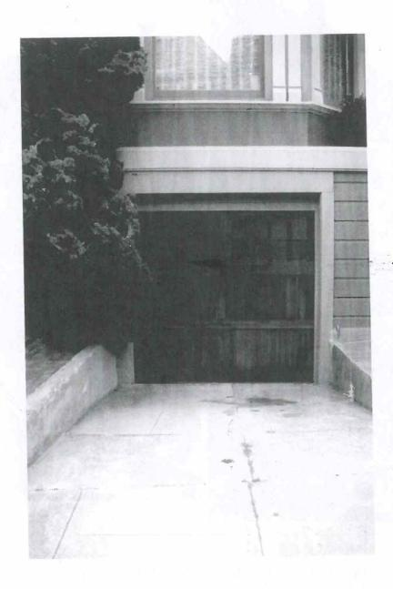
Garage door showing water damage due to slope of driveway and improper drainage. Trench drain proposed in front of garage door to collect water before it can go into the garage.
