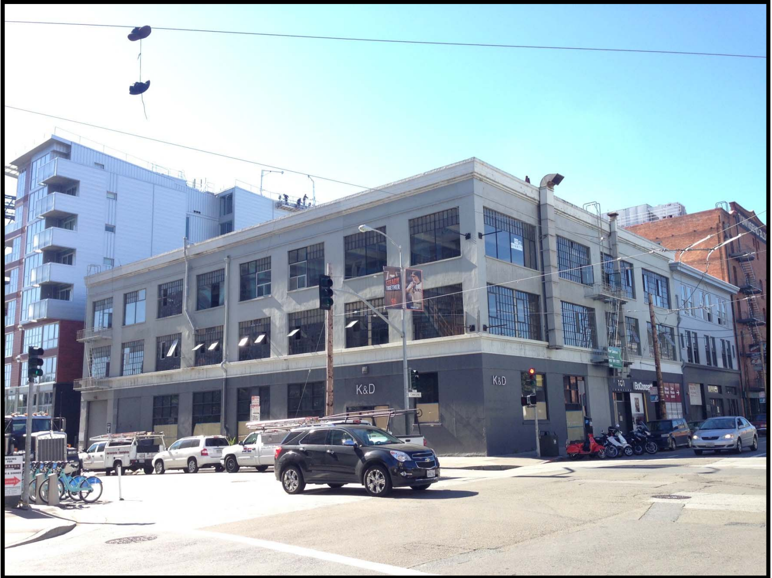
101 Townsend Street (Source: SF Planning Dept)
